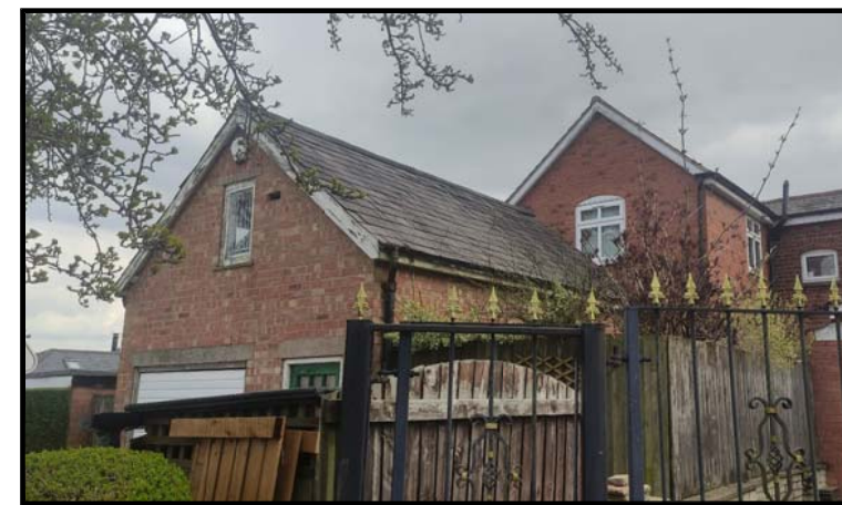
SIDE ELEVATION PHOTOGRAPH
