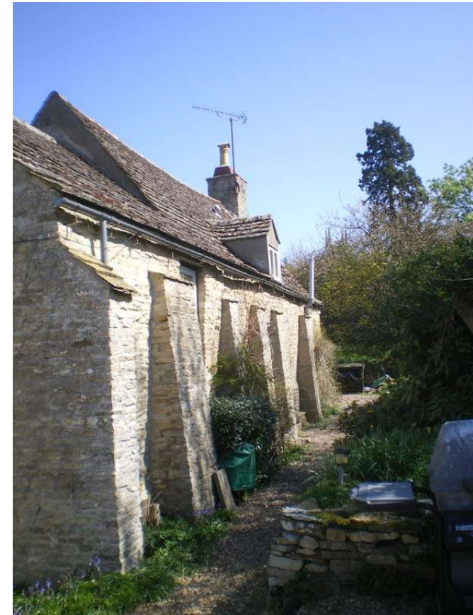
Image 2 South elevation with buttress pre extension
