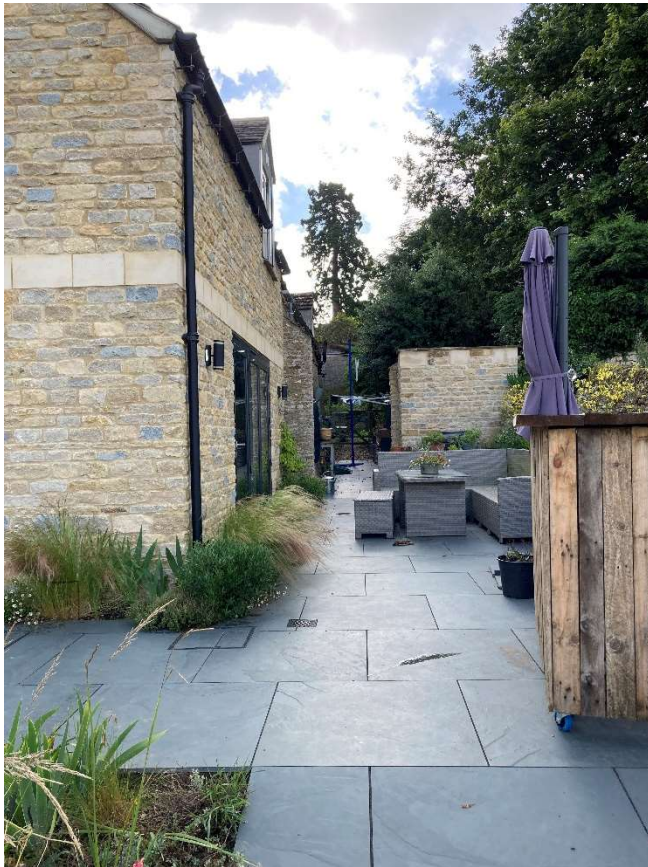
Image 1 South elevation post rear extension
