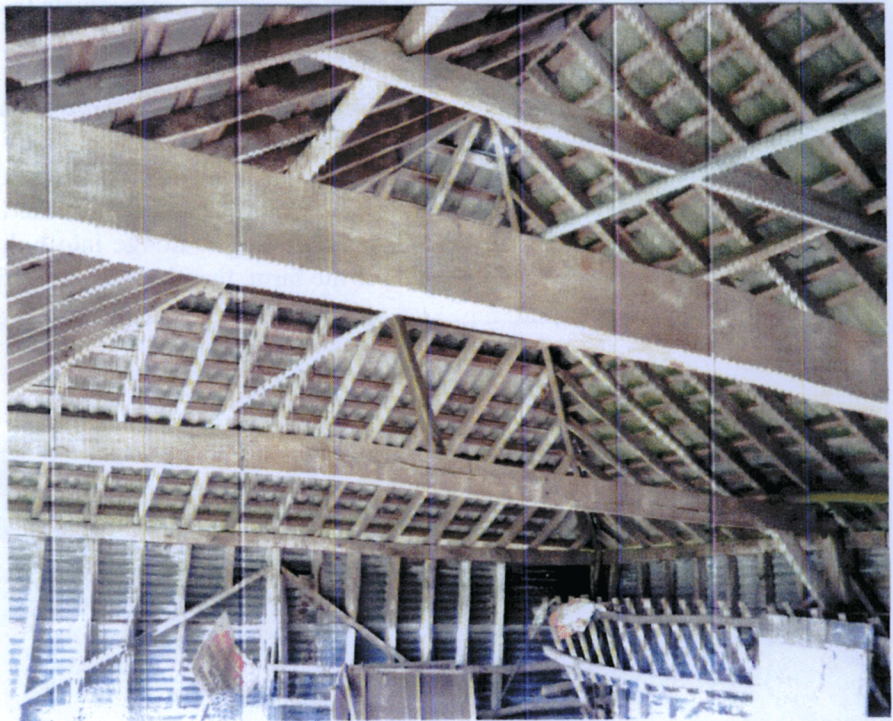
Inside the Wagon Lodge looking up at the roof structure
