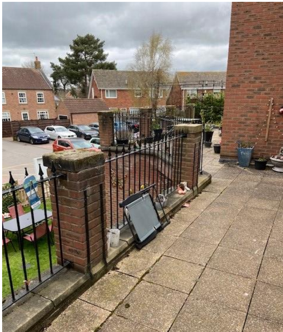
Photo 2 – View from first floor roof terrace.
