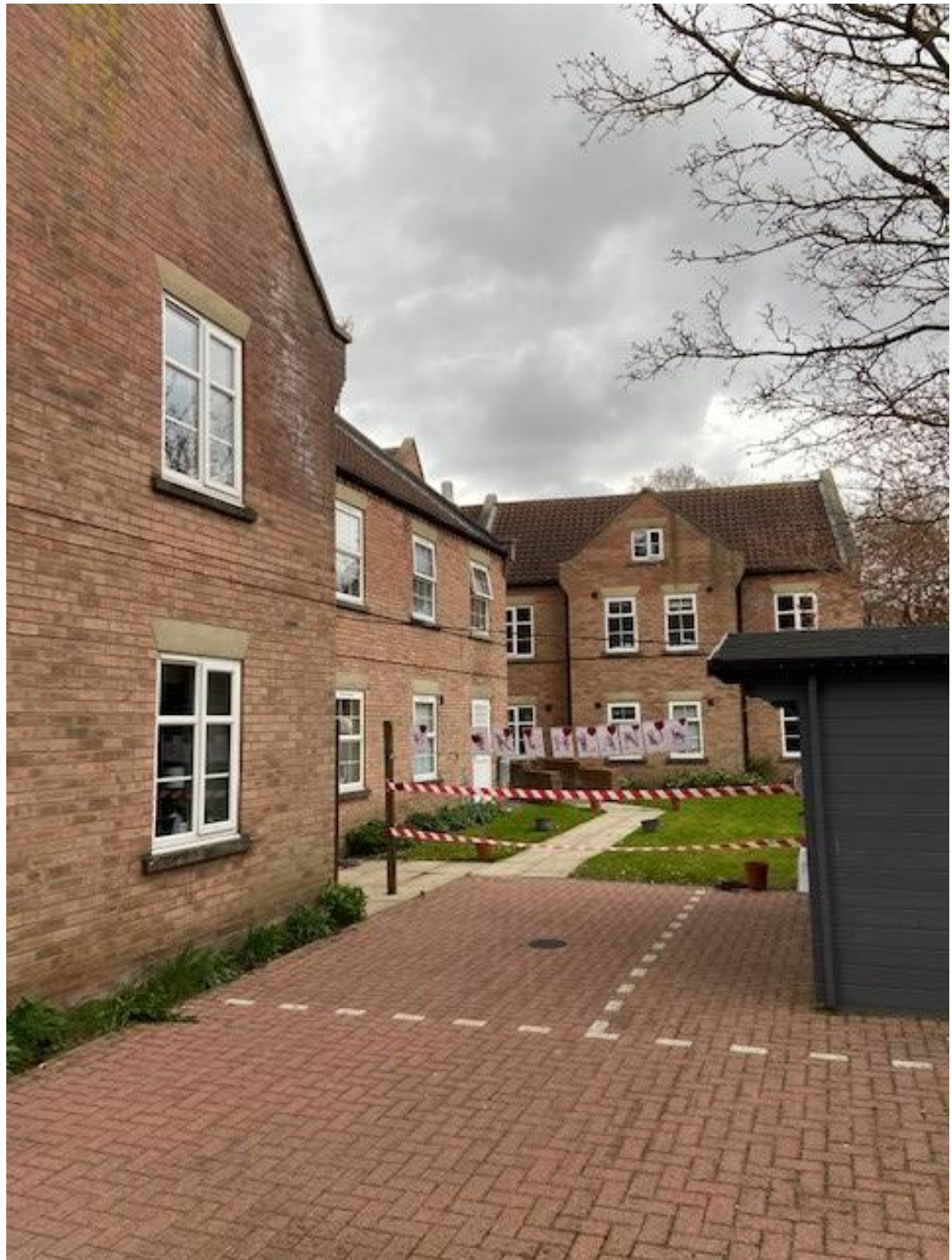
Photo 3 – Proposed side extension development area (with temporary Covid safe lounge visible). Single staff car parking space.
