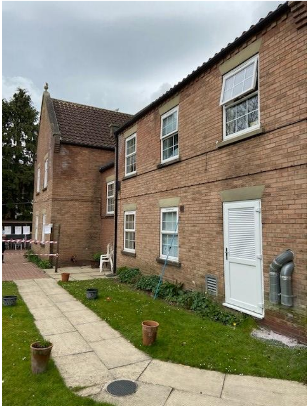
Photo 5 – View of side extension development site garden looking West.
