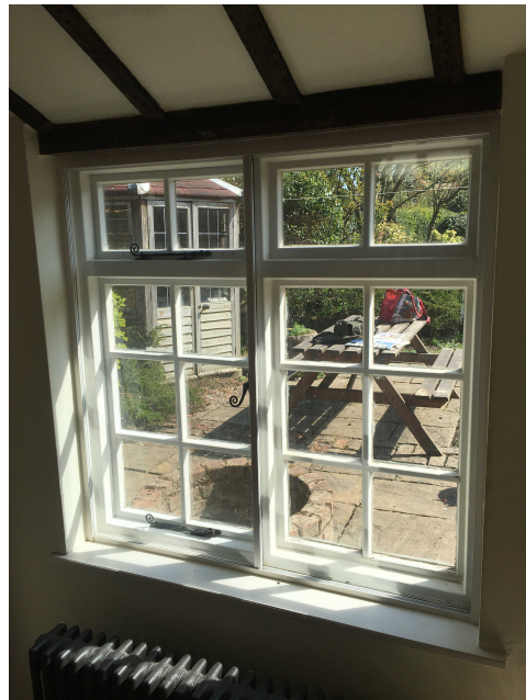
Interior view of the existing sitting room window to be retained.
