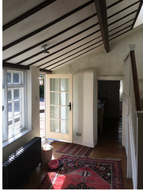
Photograph of the existing sitting room interior showing the glazed door, window, door to the kitchen and existing staircase.
