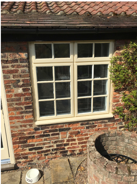
Photograph of the existing window to the sitting room to be retained. The proposed window is to be designed, fabricated and installed to match.
