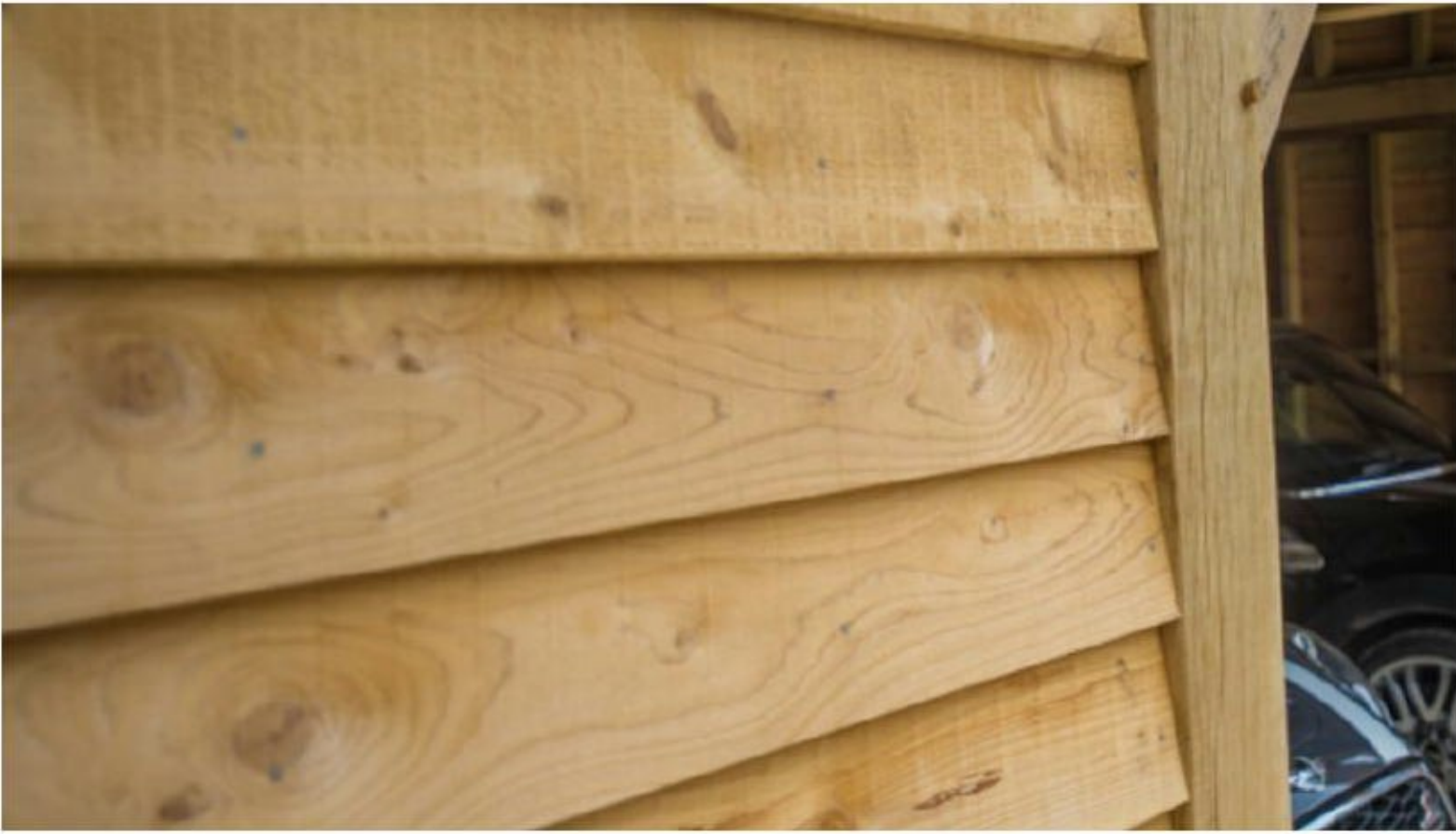
Example of horizontal timber boarding for external walls of proposed 3 Bay Cart Shed
