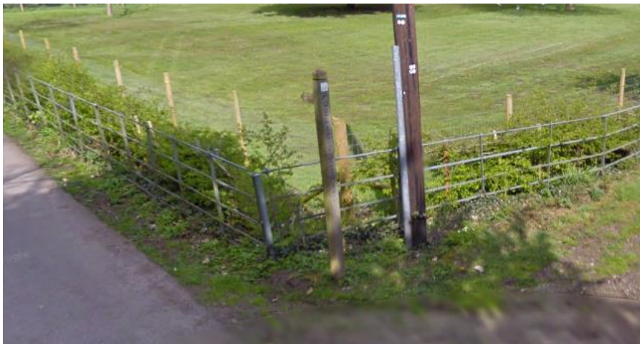
Figure 6: Galvanized Estate Fencing adjacent application site (image taken from Google Earth (c))
