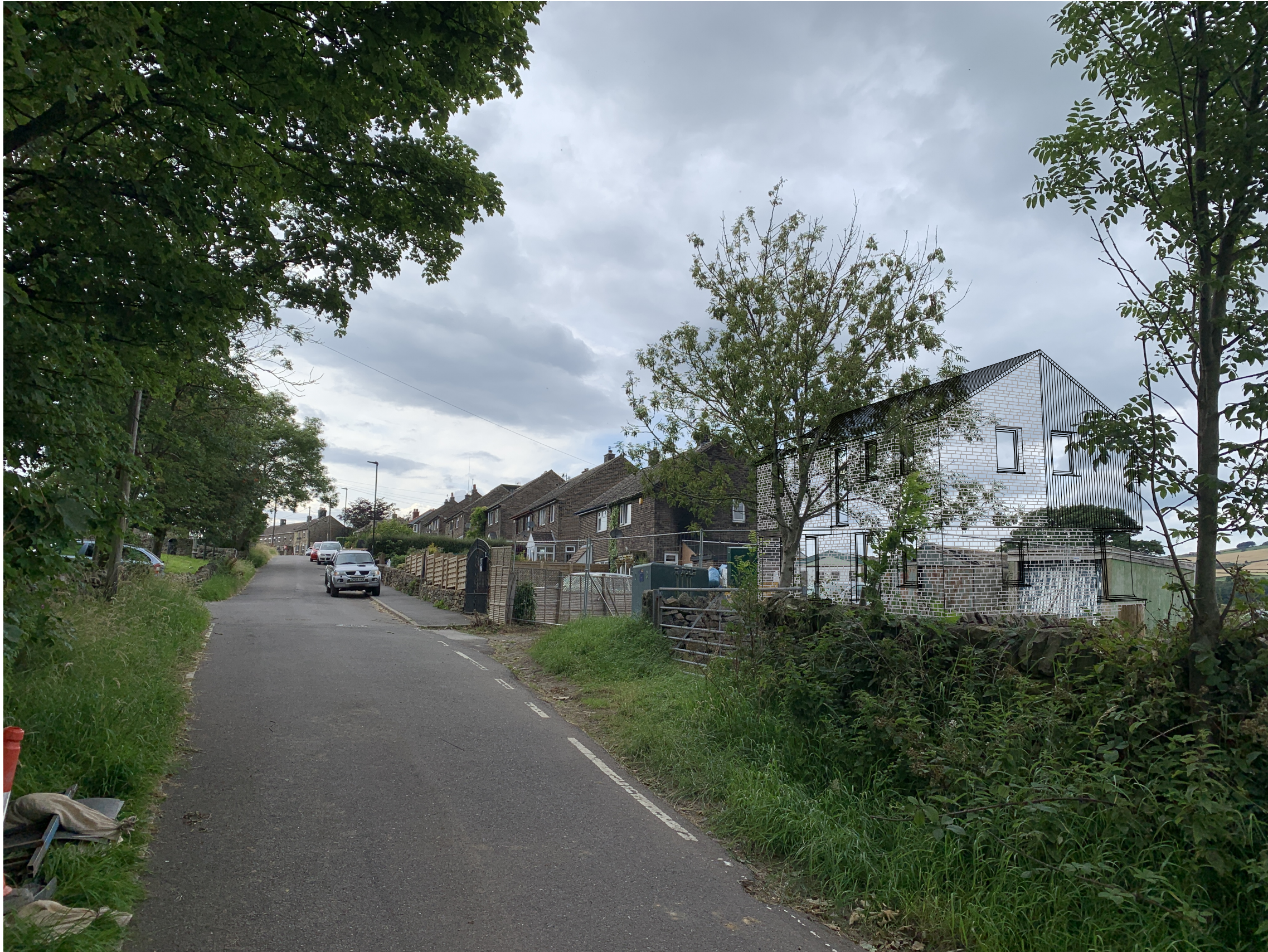
View on Uphill Approach
