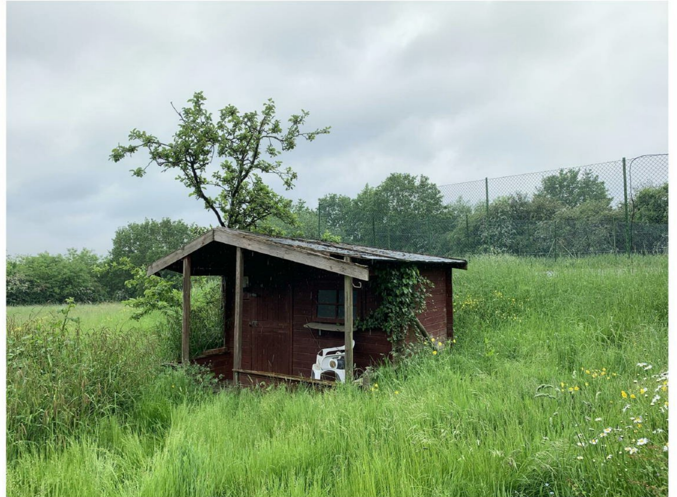
Photograph 8 – B4 shed, exhibiting negligible bat roost potential
