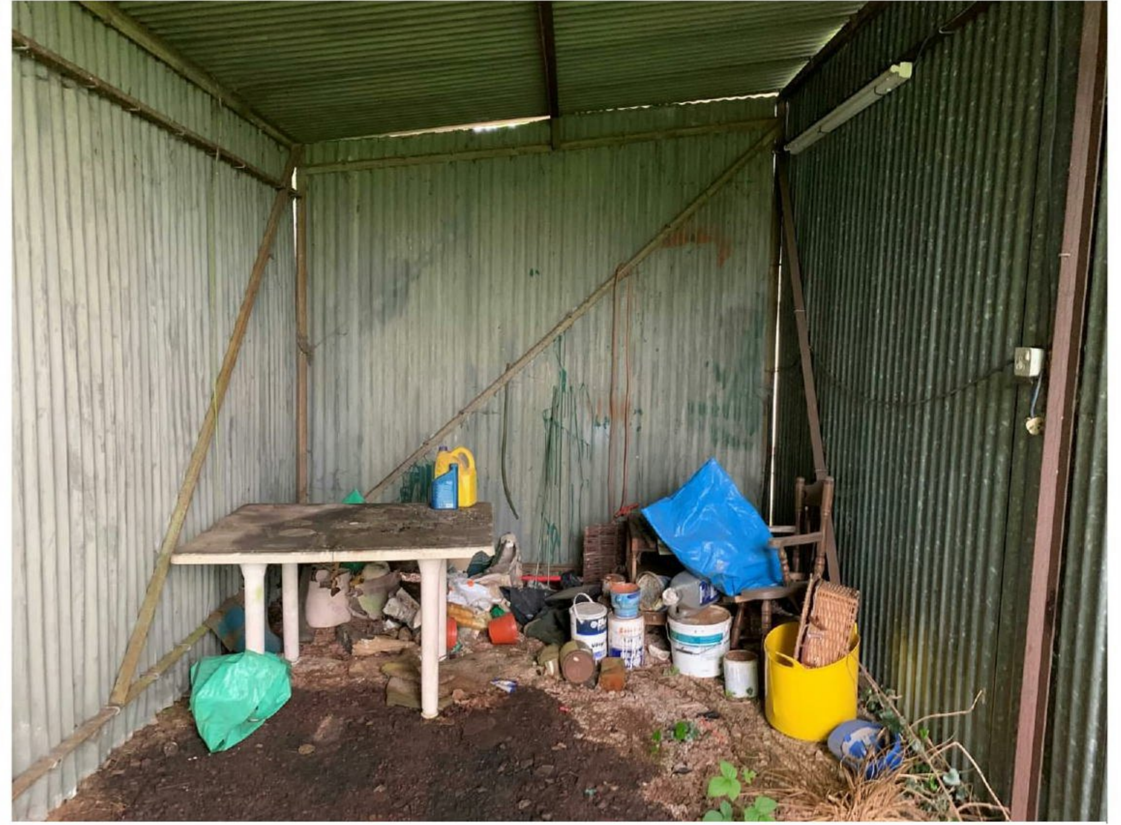
Photograph 10 – B6 metal shed exhibiting negligible bat roost potential
