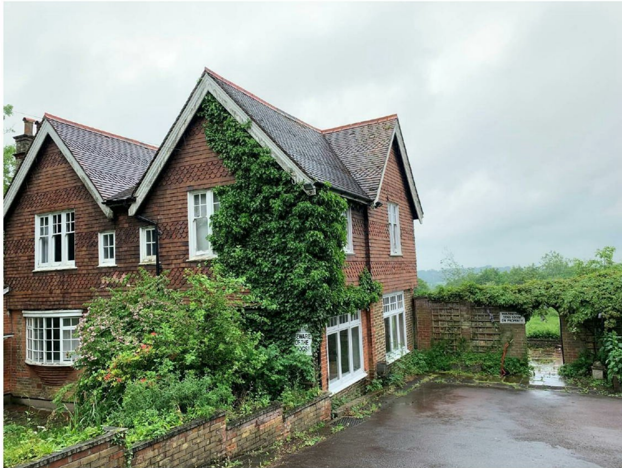
Photograph 5 – Northern and western aspect of B1 ivy coverage indicated
