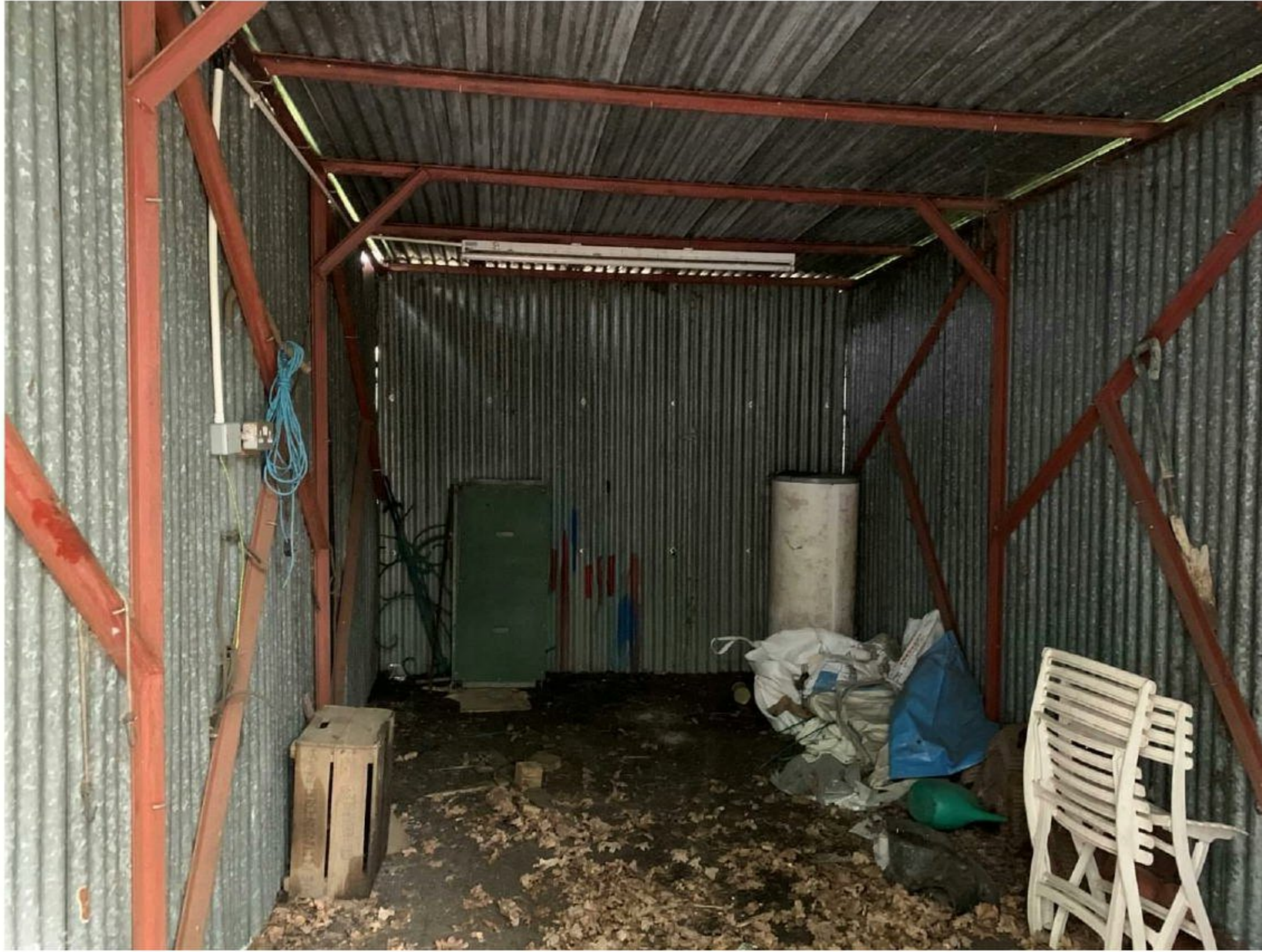
Photograph 9 – B5 metal shed exhibiting negligible bat roost potential
