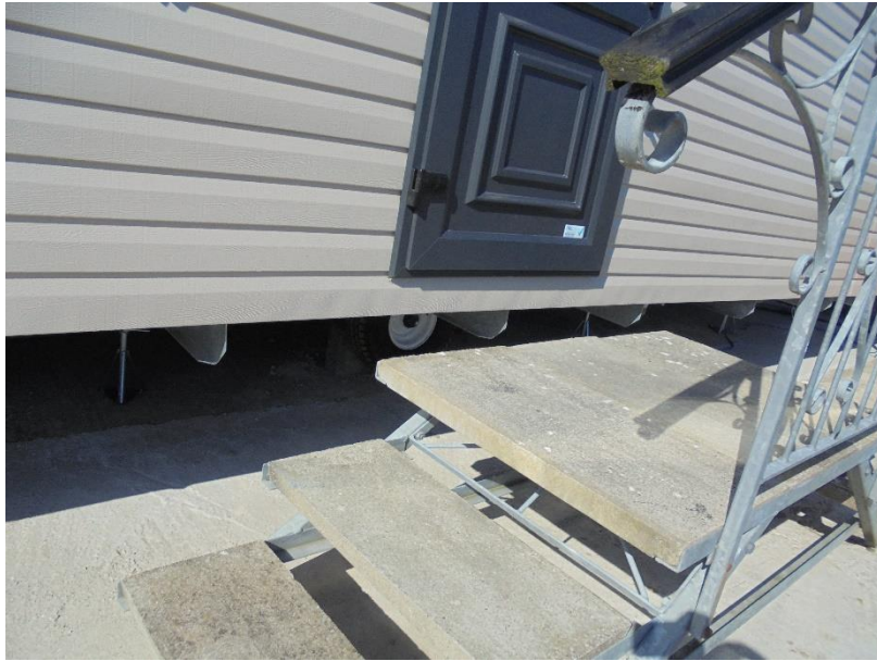
Photo 5: Example of the 0.7m freeboard on holiday homes.
