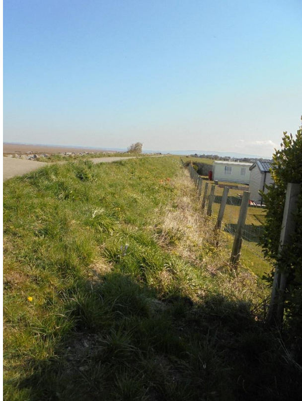
Photo 11: Embankment, path and sea defences to the North of the site.
