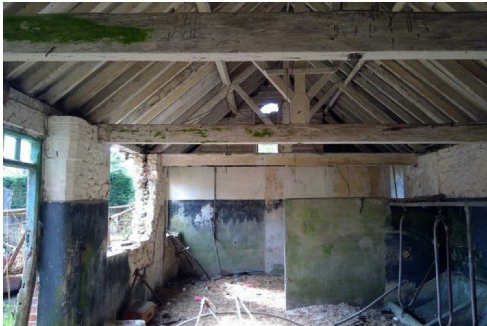
Photo 4: Interior of Building B
