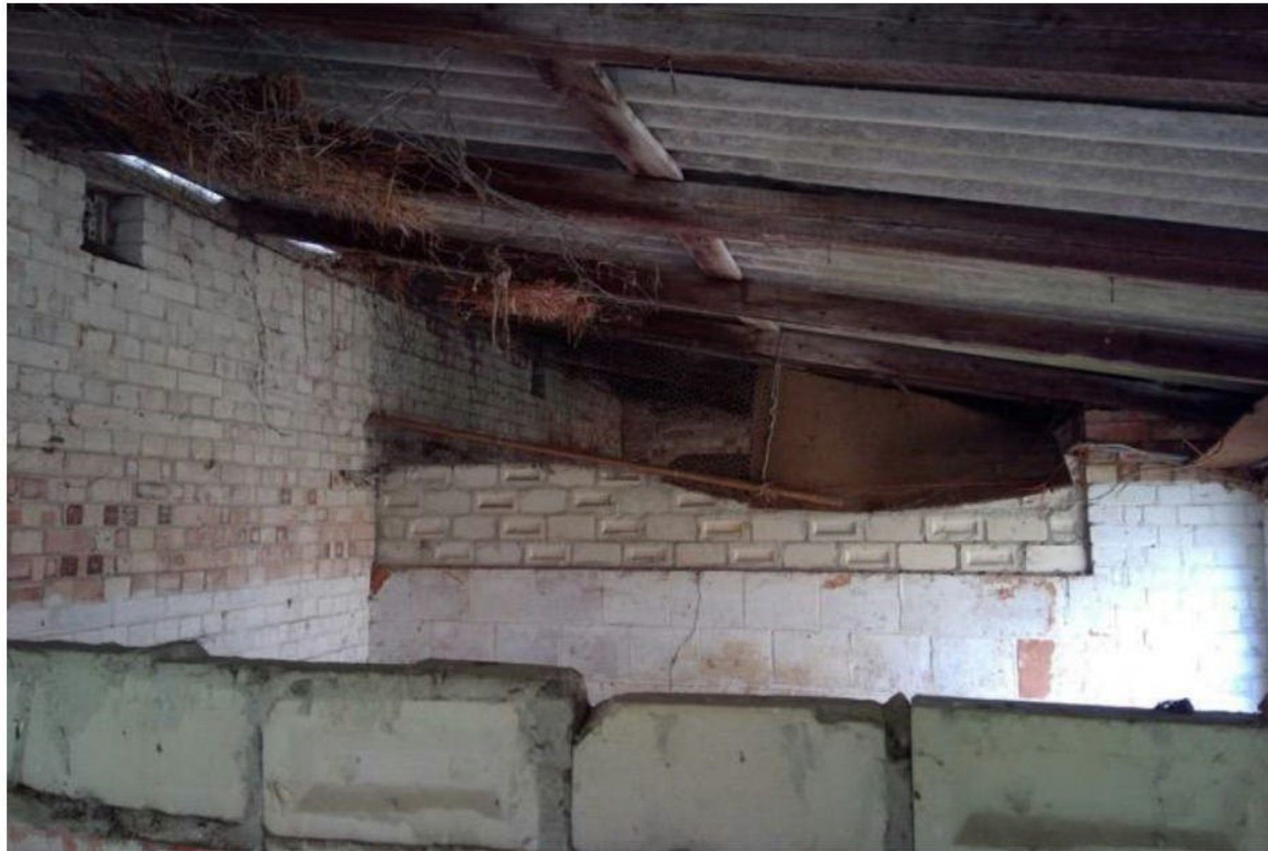
Photo 8: Interior of the stable section of building D
