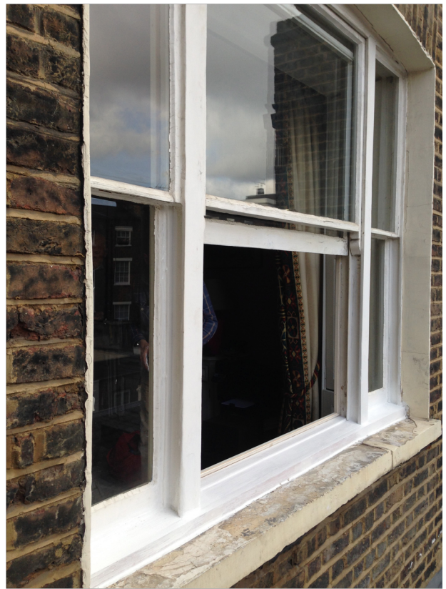
Sill replacement on a Regency - Venetian Sash Window in Belgravia W1 (Listed Grade II*)
