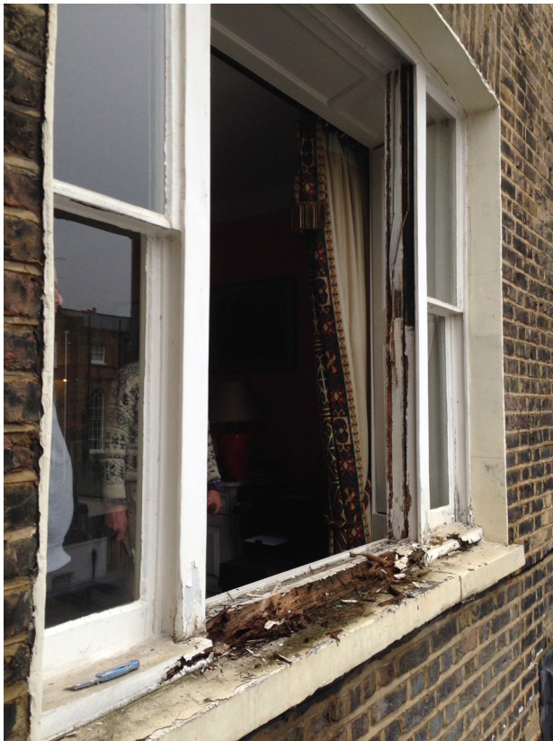
Sill replacement on a Regency - Venetian Sash Window in Belgravia W1 (Listed Grade II*)
