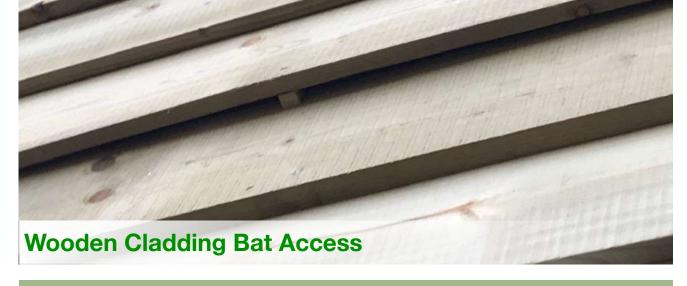
Wooden cladding features can be cheaply and easily created using materials available on site to provide a bespoke mitigation solutions for bat licence projects.
