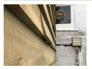
Access points can be created by pegging out small sections of wooden cladding, or by cutting out small sections at the bottom edge of the boards. When lined with bitumastic felt these create the perfect warm crevices in which birds like to nest and bats to roost.
