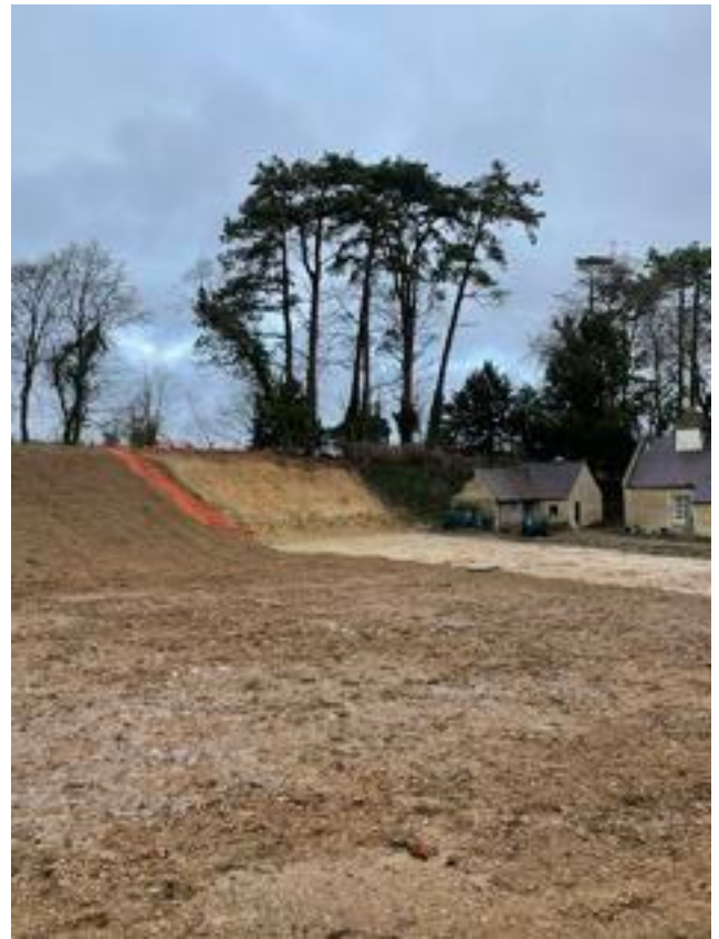
3- South-west elevation (stone outbuilding and exposed earth bank)
