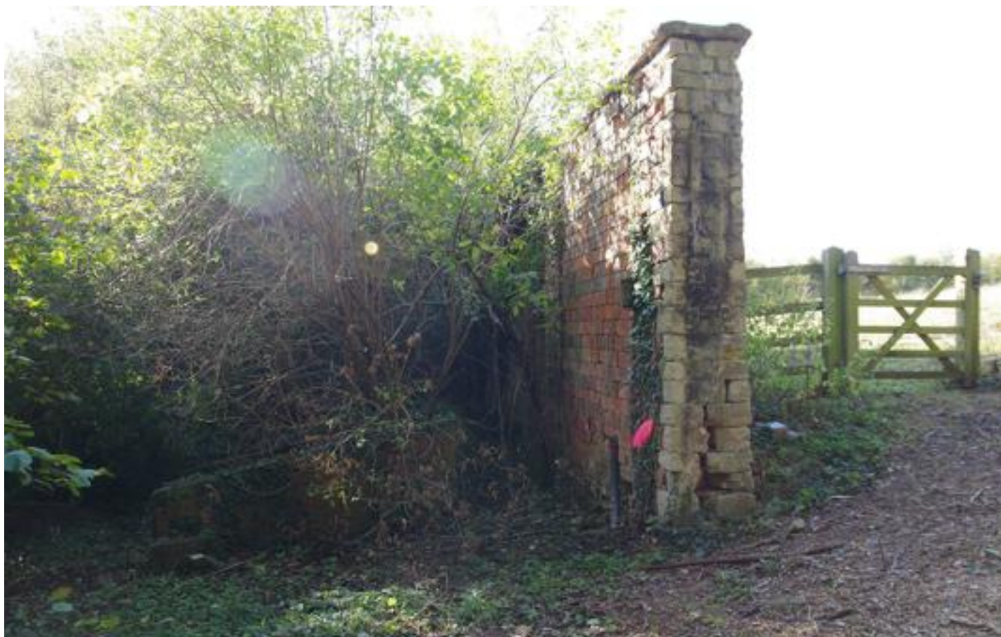
The eastern end of the northern wall of the walled garden
