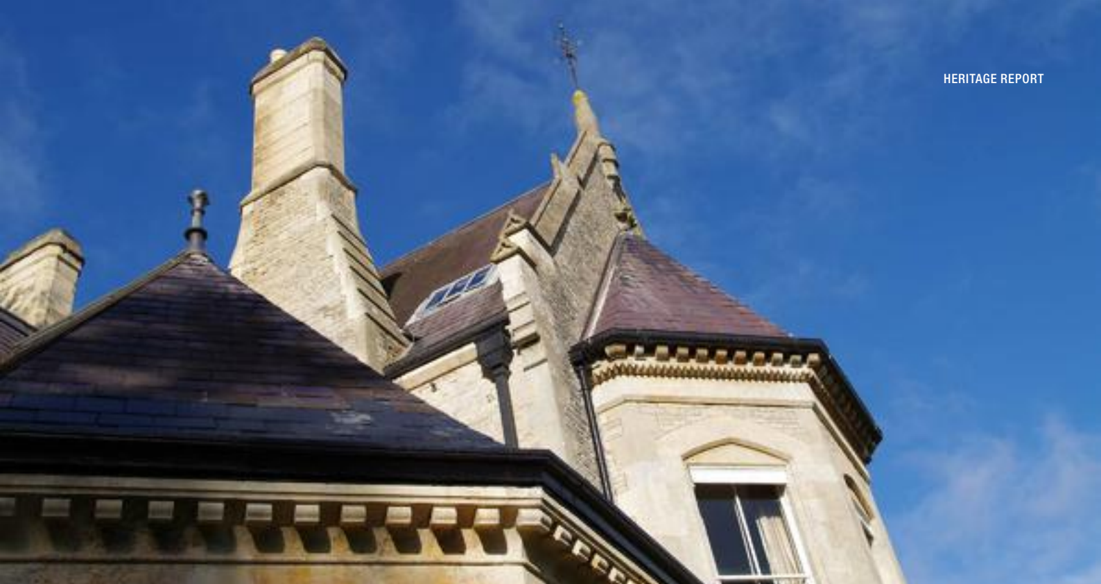
View of the c 1911-19 Library extension to the west with similar, but simpler, carved eaves detail decorative corbel and coping to the gable with iron finial, large projecting stone chimney, steep pitched gable and hipped roofs.
