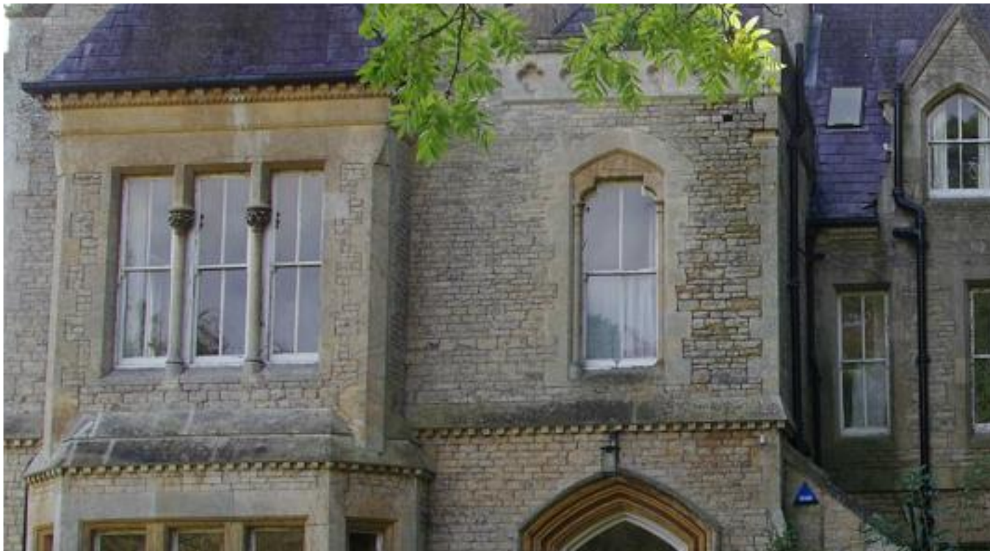
East elevation showing range of Gothic architectural detailing – deeply moulded arched entrance to porch, arched window over with capitals to architraves, quatrefoil parapet detail to top of porch, dentil string course, foliate capitals to the two mullions of the first floor projecting bay window, carved details to eaves, steep pitched hipped roof
