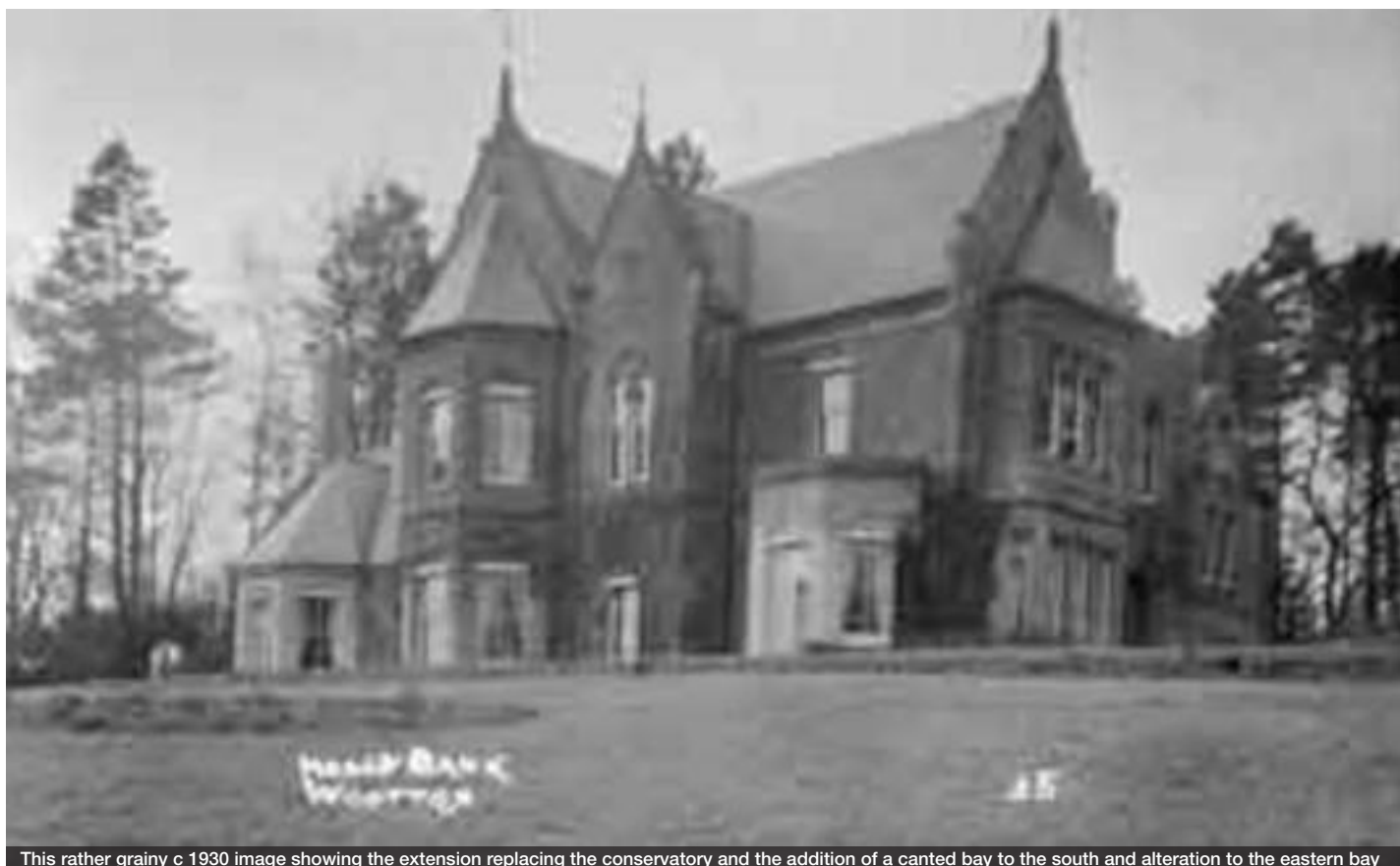
This rather grainy c 1930 image showing the extension replacing the conservatory and the addition of a canted bay to the south and alteration to the eastern bay
