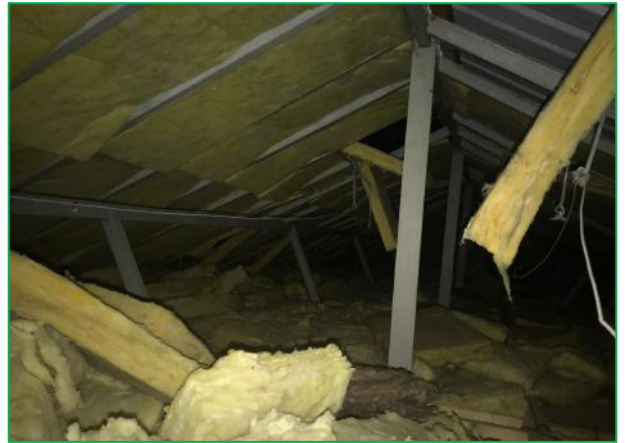
A loft space in Structure 2
