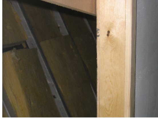
Interior of the building identifying the boxing in of the metal frame of the original glasshouse structure
