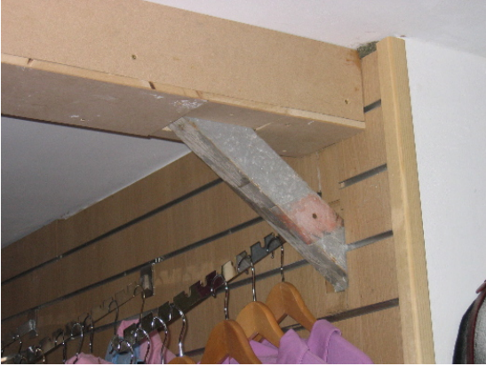
Interior of the building identifying the boxing in of the metal frame of the original glasshouse structure
