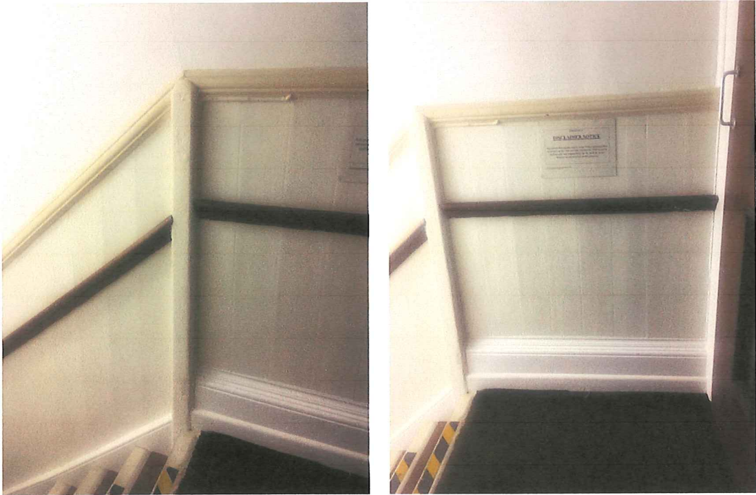
Figs 9 (a) and 9 (b) - Panelling to side of stairs at top landing.
