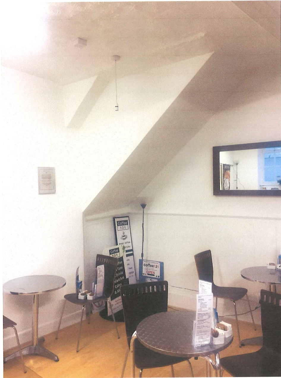
Fig 3 - Underside of Stairs
