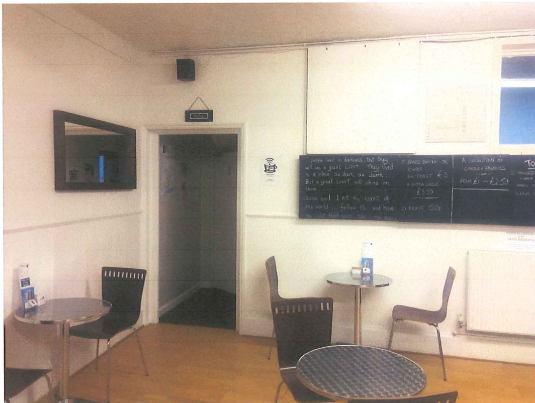
Fig 15 - Doorway D.5. in Cafe.
