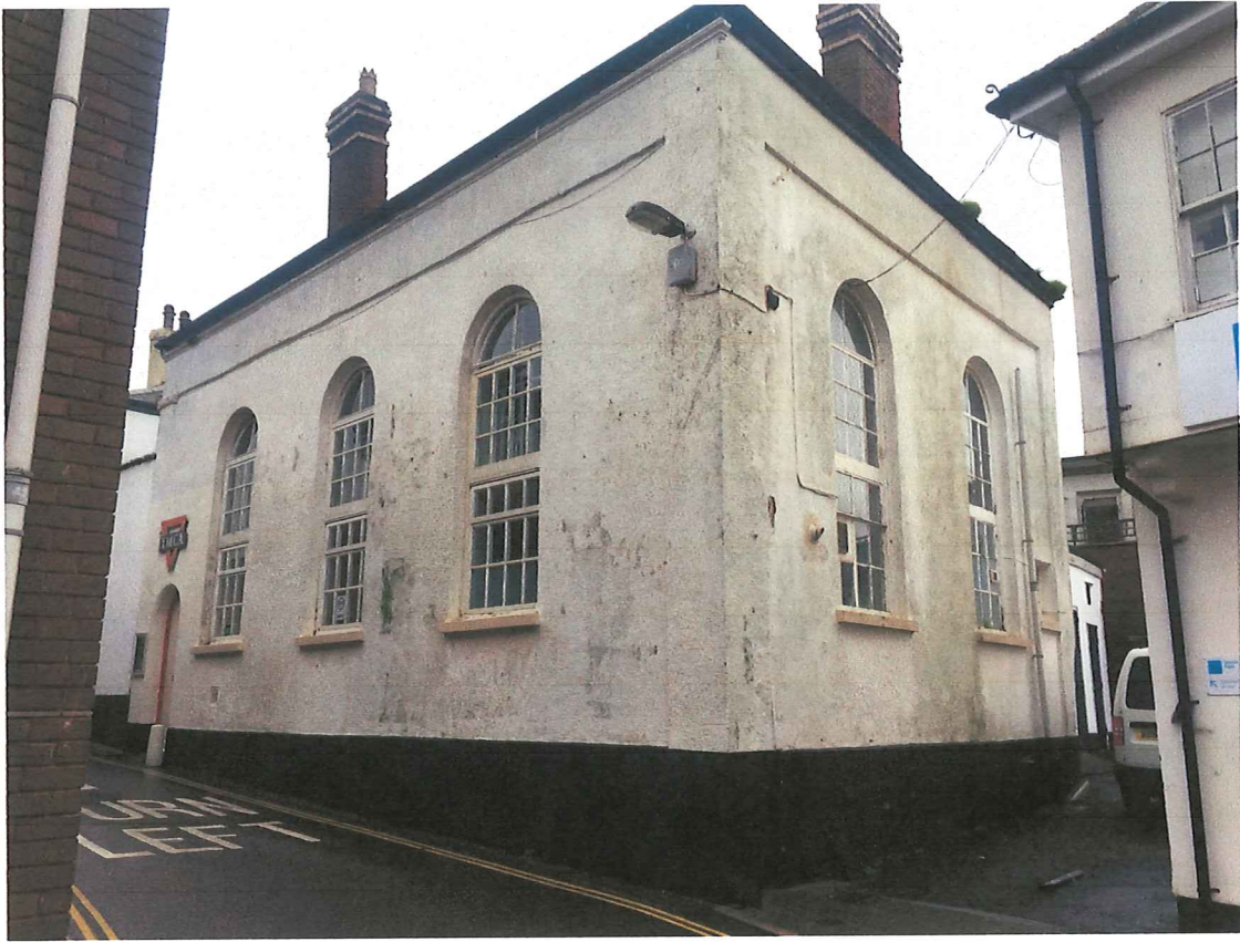
Fig 1 - Two Main External Elevations.
