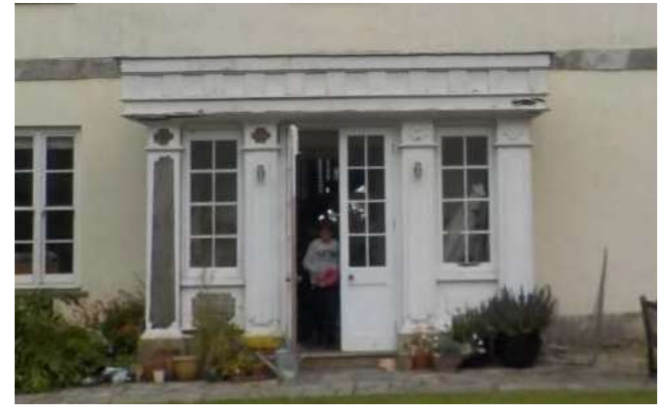
Fig 14. - Archive photograph showing porch on front of building
