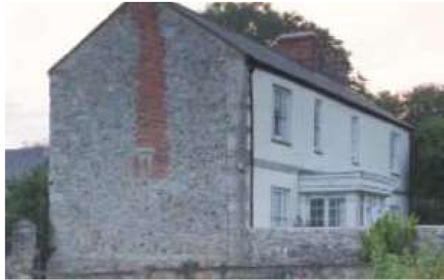
Fig 13. - Archive photograph showing porch on front of building
