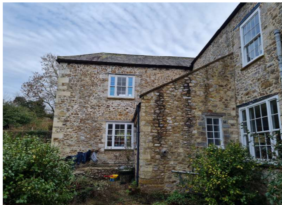
Fig 22. North elevation of farmhouse and east elevation of existing rear projection showing location of proposed 2 storey extension, in lieu of existing single storey extension. Note modern windows and window openings.
