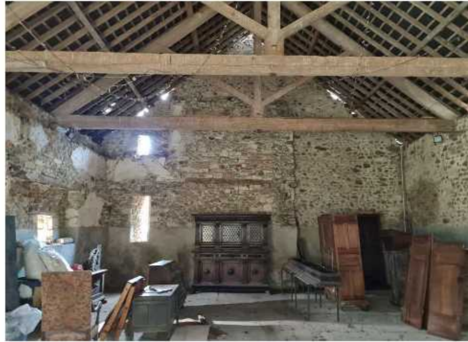
Fig 13. Existing barn looking west towards western gable and location of proposed reinstated fireplace.
