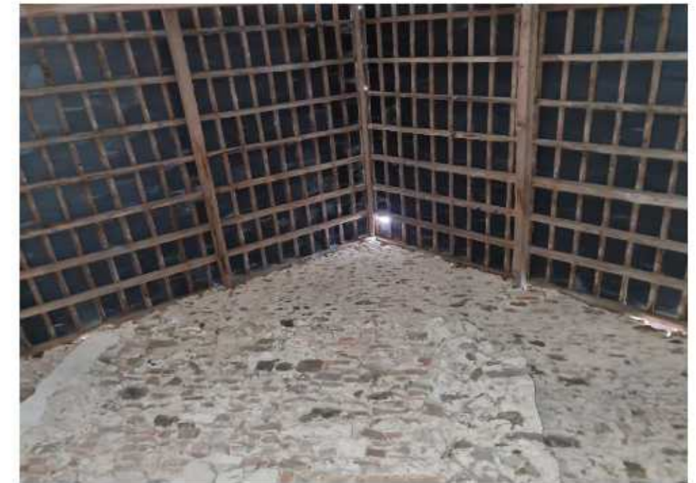
Fig 16. Detail photograph of internal side of western gable of barn looking up to roof.
