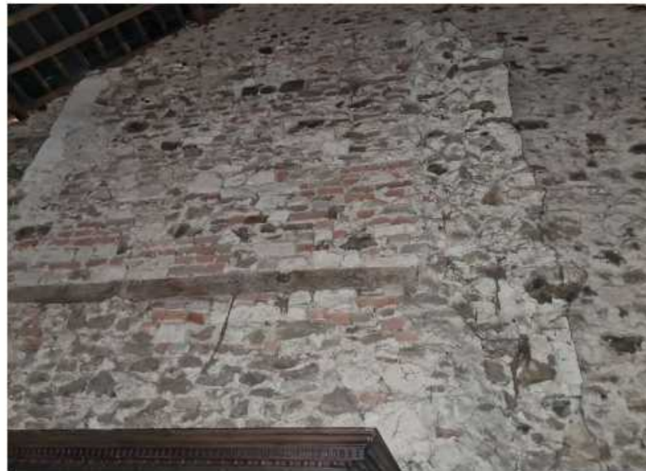
Fig 15. Detail photograph of internal side of western gable of barn.
