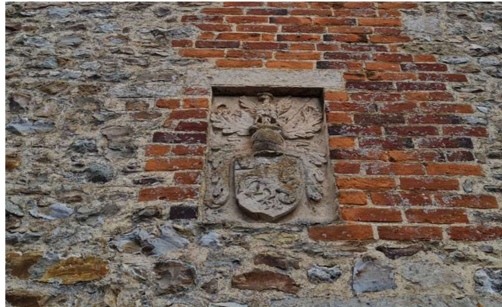
Fig 5. - Drakes of Ashe Coat of Arms set in west gable of farmhouse.
