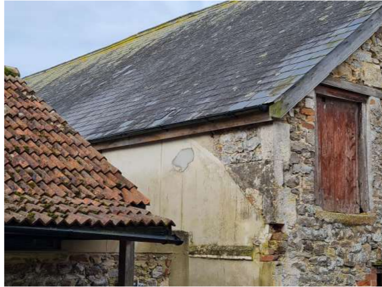
Fig 17. Photo showing 'tide mark' of former roof of dairy barn connecting with the manor barn.
