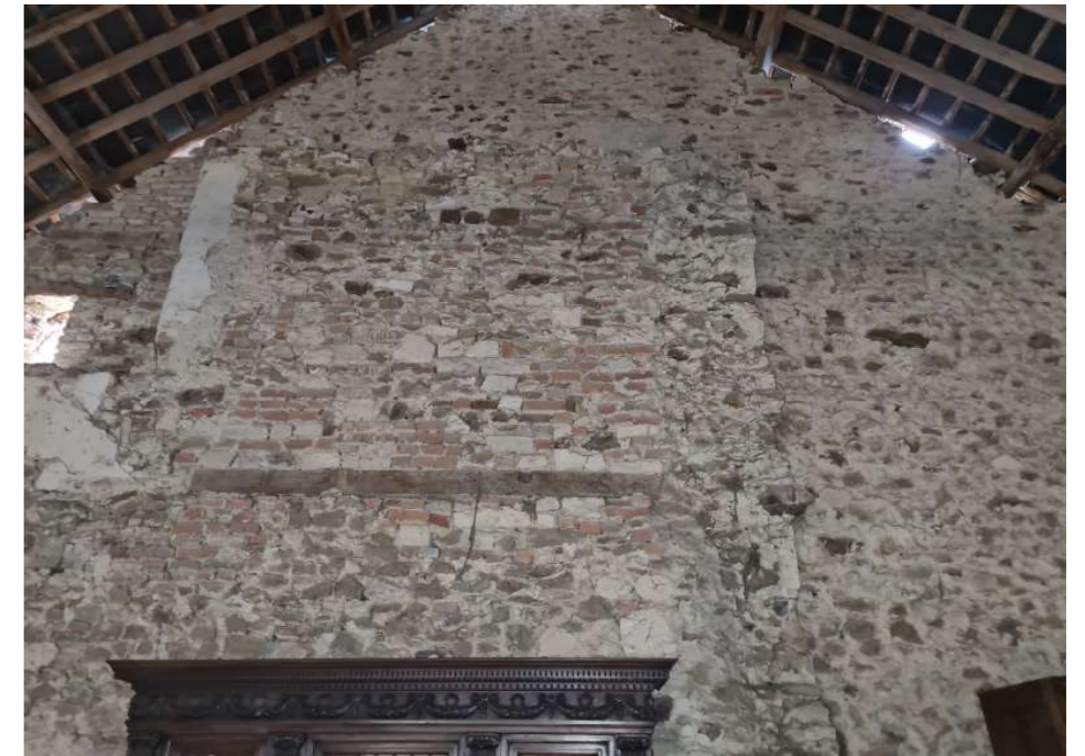
Fig 14. Detail photograph of internal side of western gable of barn.
