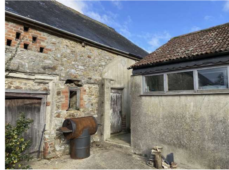
Fig 18. Photo showing 'tide mark' of former roof of dairy barn connecting with the manor barn as viewed from southern courtyard.
