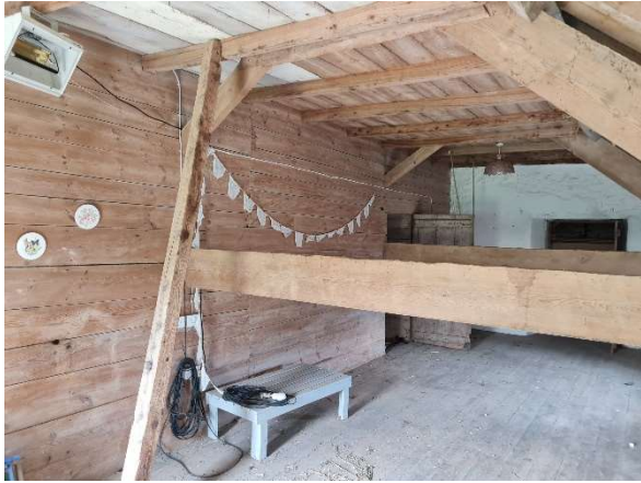
Existing first floor showing low level of truss.
