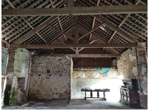
Roof structure over barn
