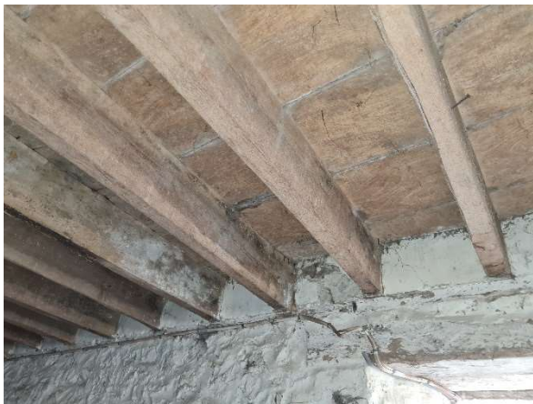
Existing first floor structure
