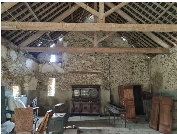
Interior view of west gable
