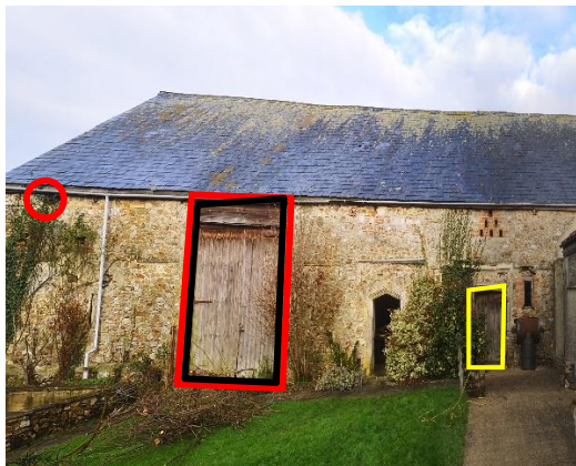
Figure 12. Locations of the emerging common pipistrelle bats (red), serotines (black) and lesser horseshoe (yellow) from the southern elevation of the barn
