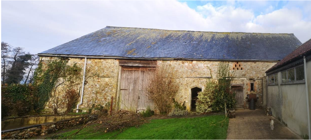
Figure 5. The southern elevation of the Manor Barn
