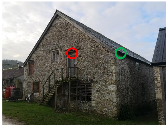
Figure 13. Location of the emerging common pipistrelle bats (red) and Natterer's bat (green) from the eastern and northern elevation of the barn
