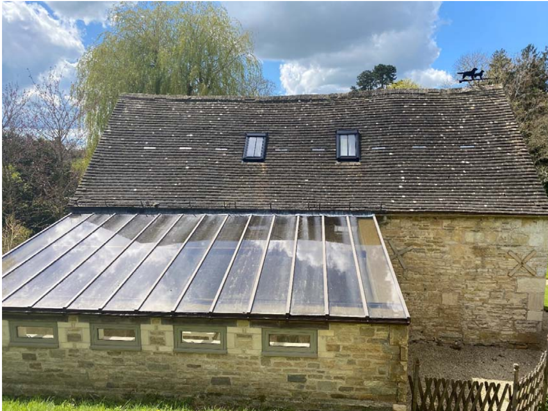
Figure 4: East elevation of outbuilding
