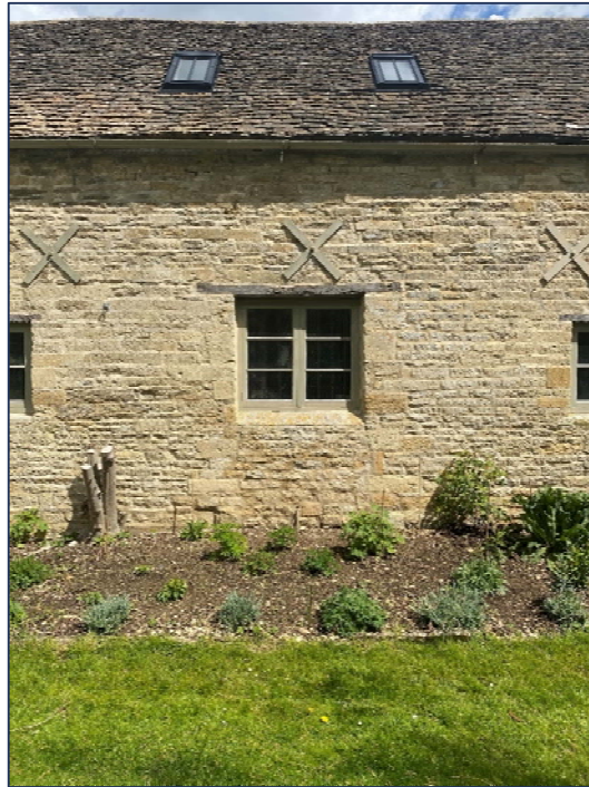
Figure 7: Western elevation of outbuilding
