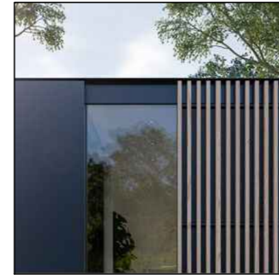
MATTE BLACK ALUMINIUM CLADDING AND GLAZING FRAMES
