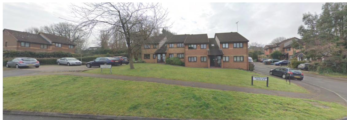
Figure 6 Apartments 54-58 Richfield road forming a terrace. View from Richfield road roundabout towards Richards close
