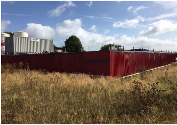
Typical Site Hoarding to Compound
