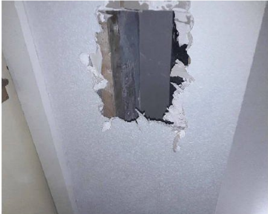
31 (24 Living Room) Beyond plaster to plasterboard wall
