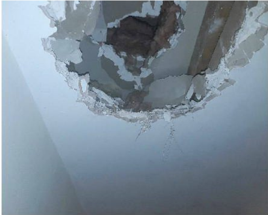
39 (33 Hallway) Beyond plaster to plasterboard wall
