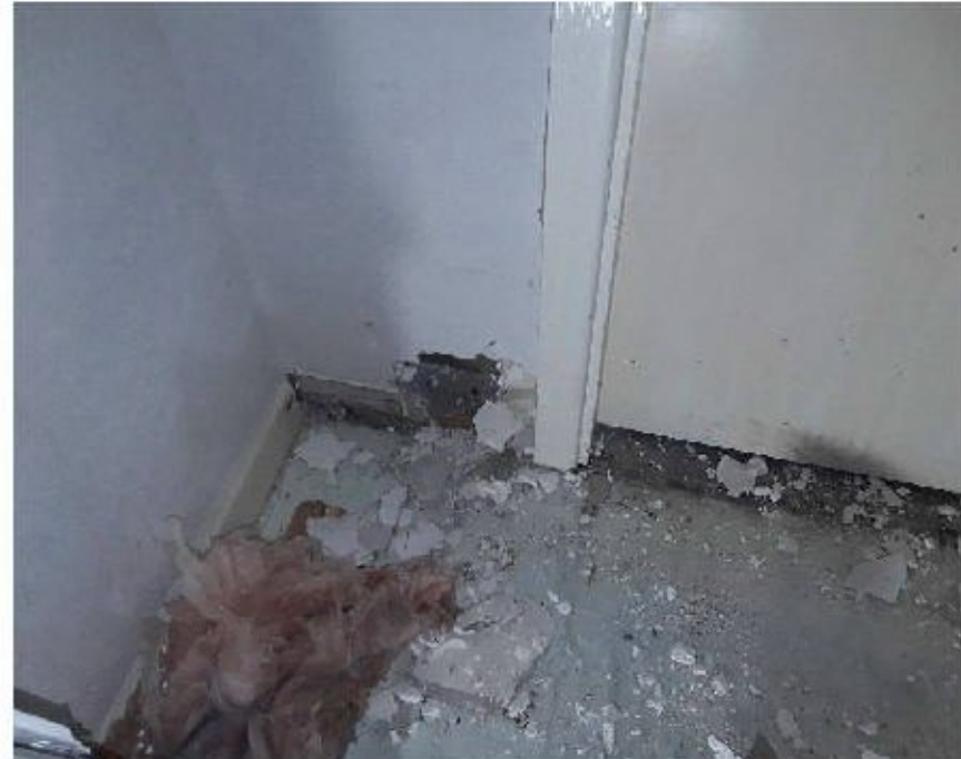
32 (25 Hallway) Beyond plaster to plasterboard cladding to beam
