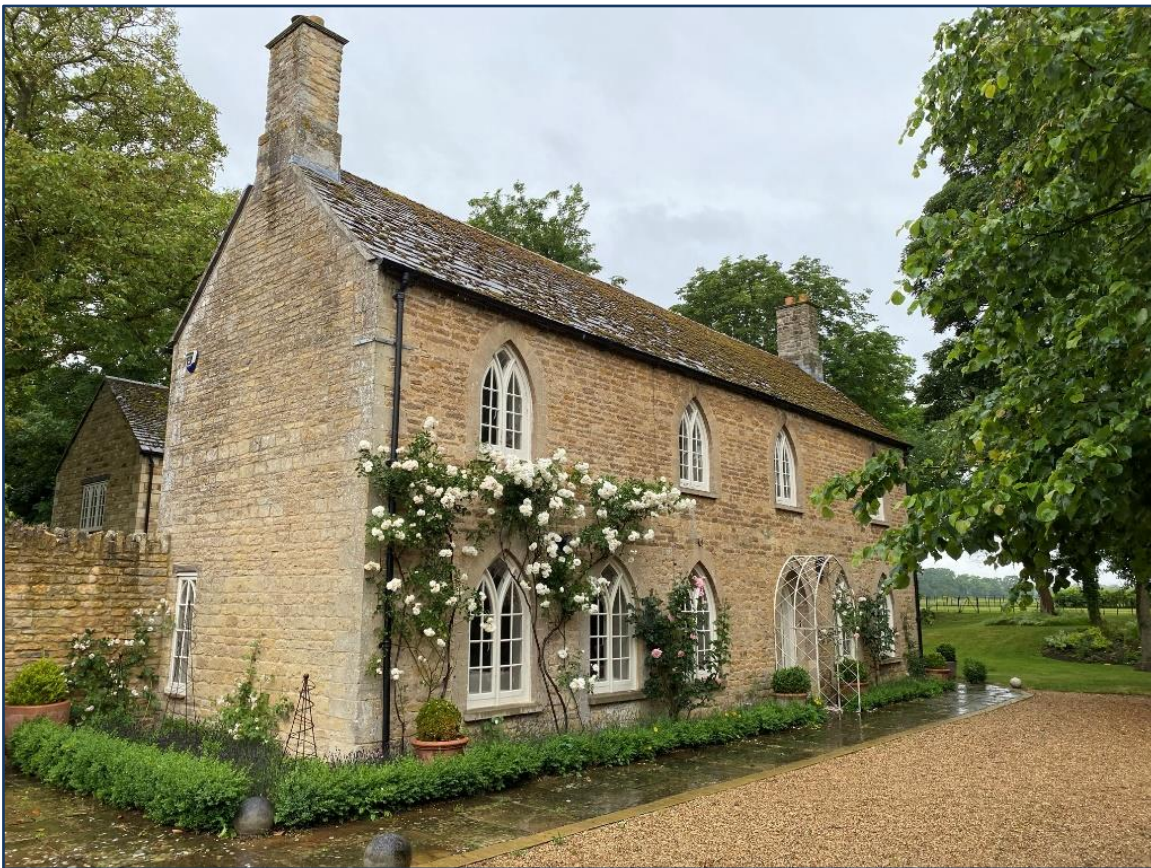
Fig. 1 – Principal / east elevation
