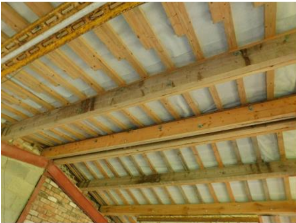
PHOTO 17 Underside of Garage Roof
