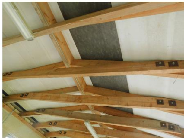
PHOTO 23 Underside of Northern Roof
