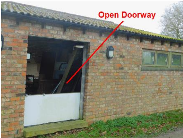
PHOTO 3 Open Doorway in Eastern Elevation
