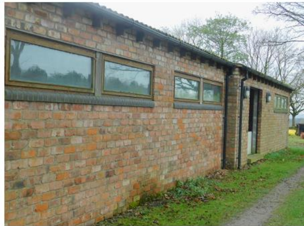
PHOTO 4 View Along South-western Elevation
