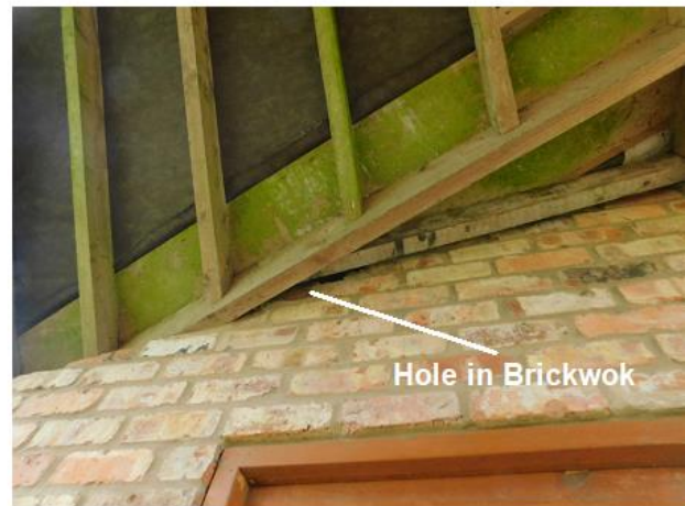
PHOTO 22 View of Part Archway Roof
