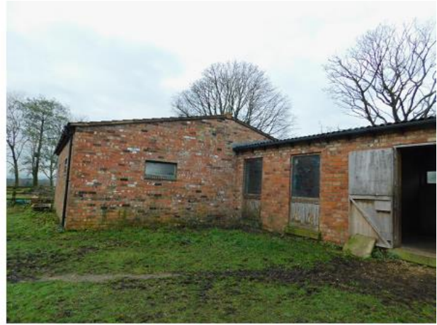
PHOTO 14 Northern Elevation of Garage
