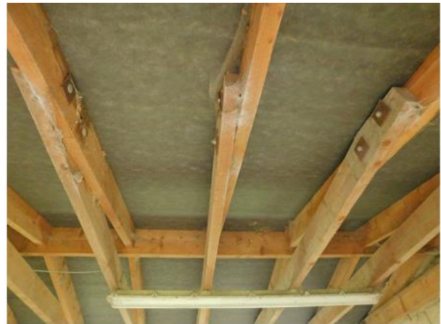
PHOTO 20 Underside of Stables Roof
