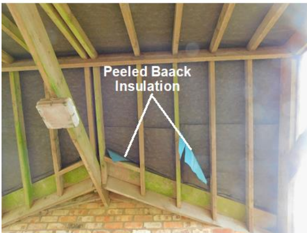
PHOTO 21 Underside of Archway Roof
