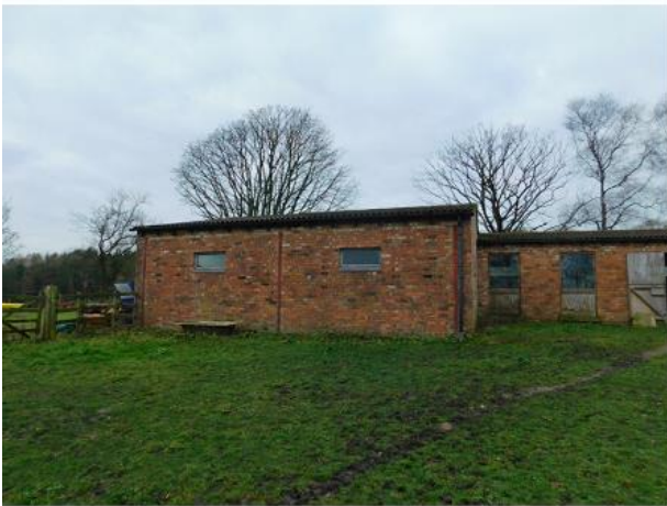
PHOTO 15 Eastern Elevation of Garage
