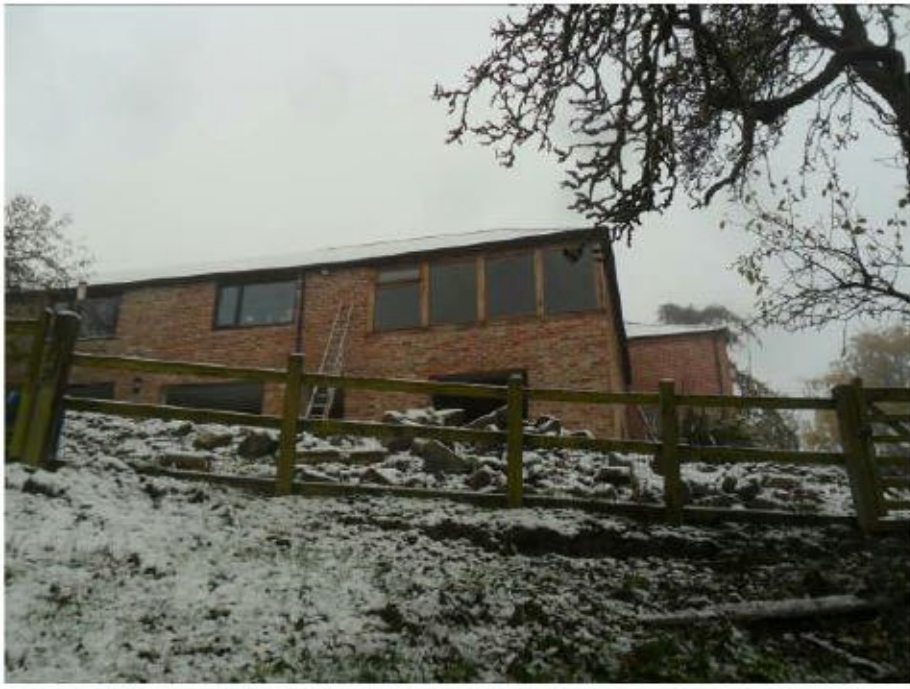
Southern aspect of extension
