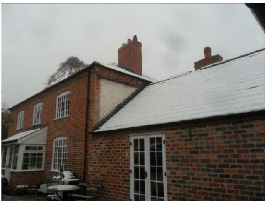
Extension abutting south of house
