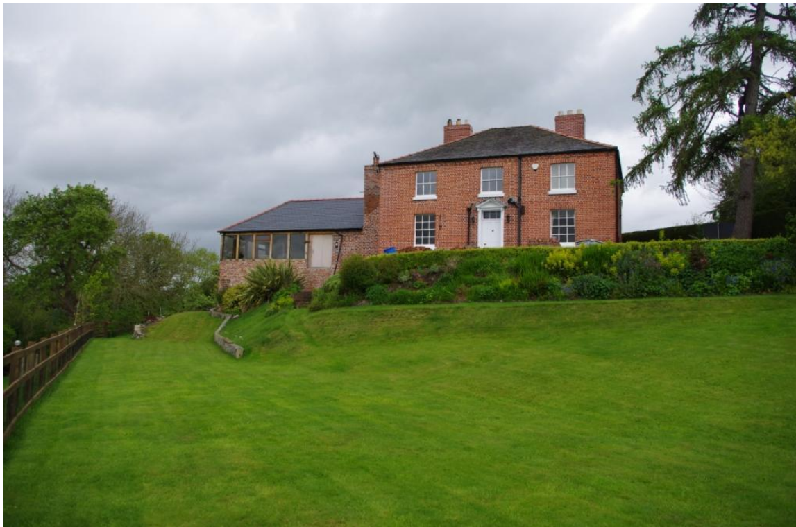
Figure 5 Principal Elevation (Looking West – North West).
