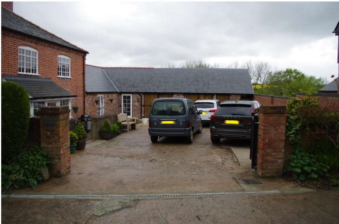
Figure 8 Outbuilding (Looking South West).
