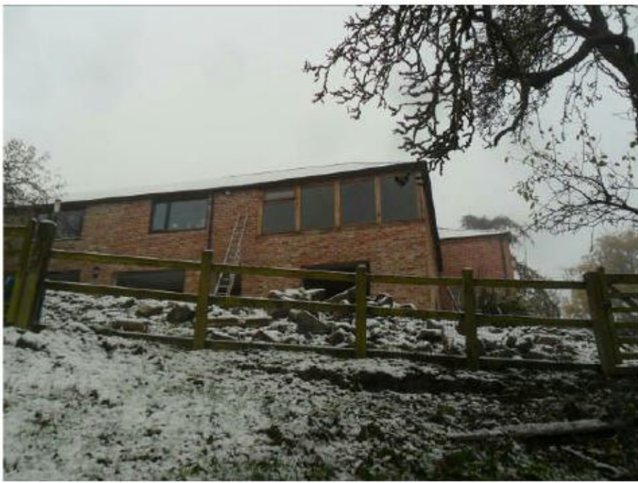
Southern aspect of extension
