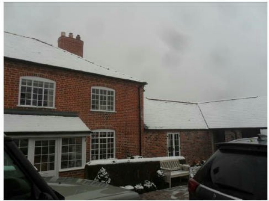
Western aspect of house & extension
