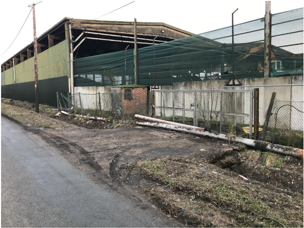
E5 – now blocked entrance. Concrete to roadside in existence
