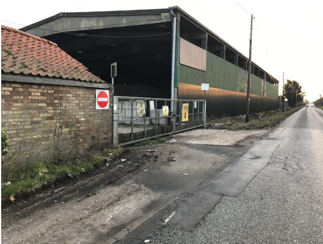
E4 – Emergency Access. Concrete to road
