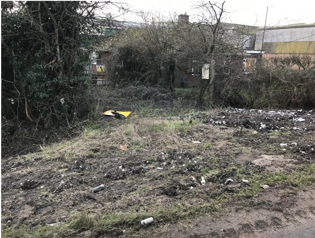
E2 – covered in overgrowth and soil. Can see was once a gate but only by looking closely.
