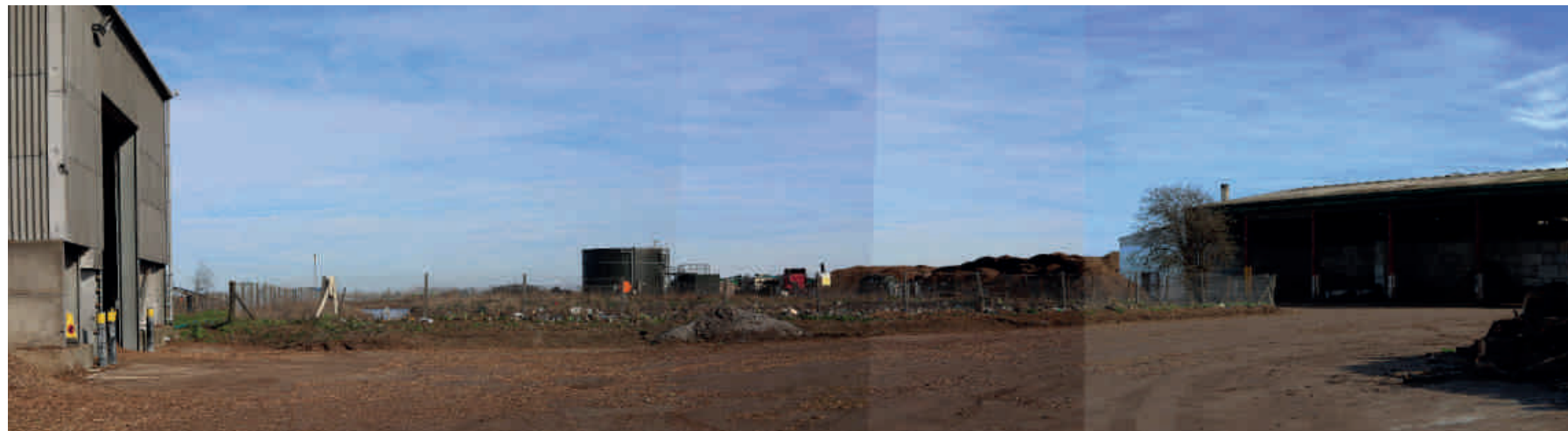
B: View Looking North over one of the Lagoons, the Compost and Waste Transfer Building is to the Left (Building No.20) and the Biomass Boiler and Finished Dry Product Storage is to the Right (Building No.21)
