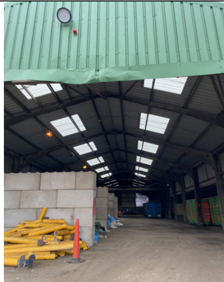
Looking through waste processing area to Structure 2
