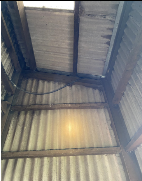
Internal void at far end of Structure 2
