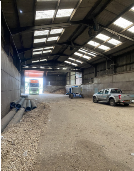
Interior of Structure 2
