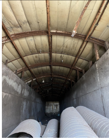
Interior of one of fabric roofed tunnels.
