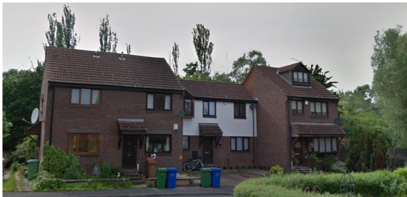
Fig.1 – Existing terrace group with the application site on the right hand side of the image.
