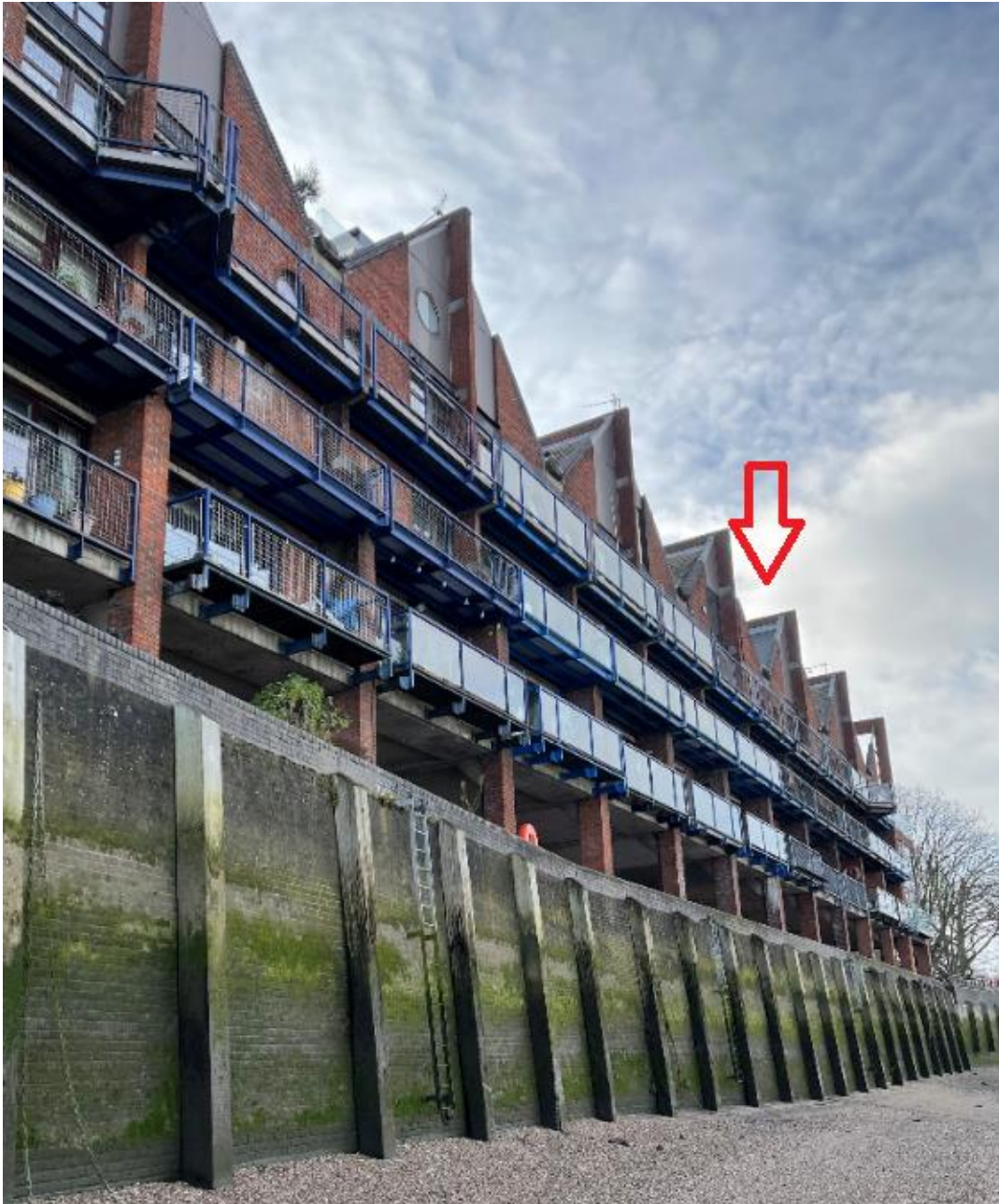
9 Kings Stairs Close (arrowed in red) – North Elevation
