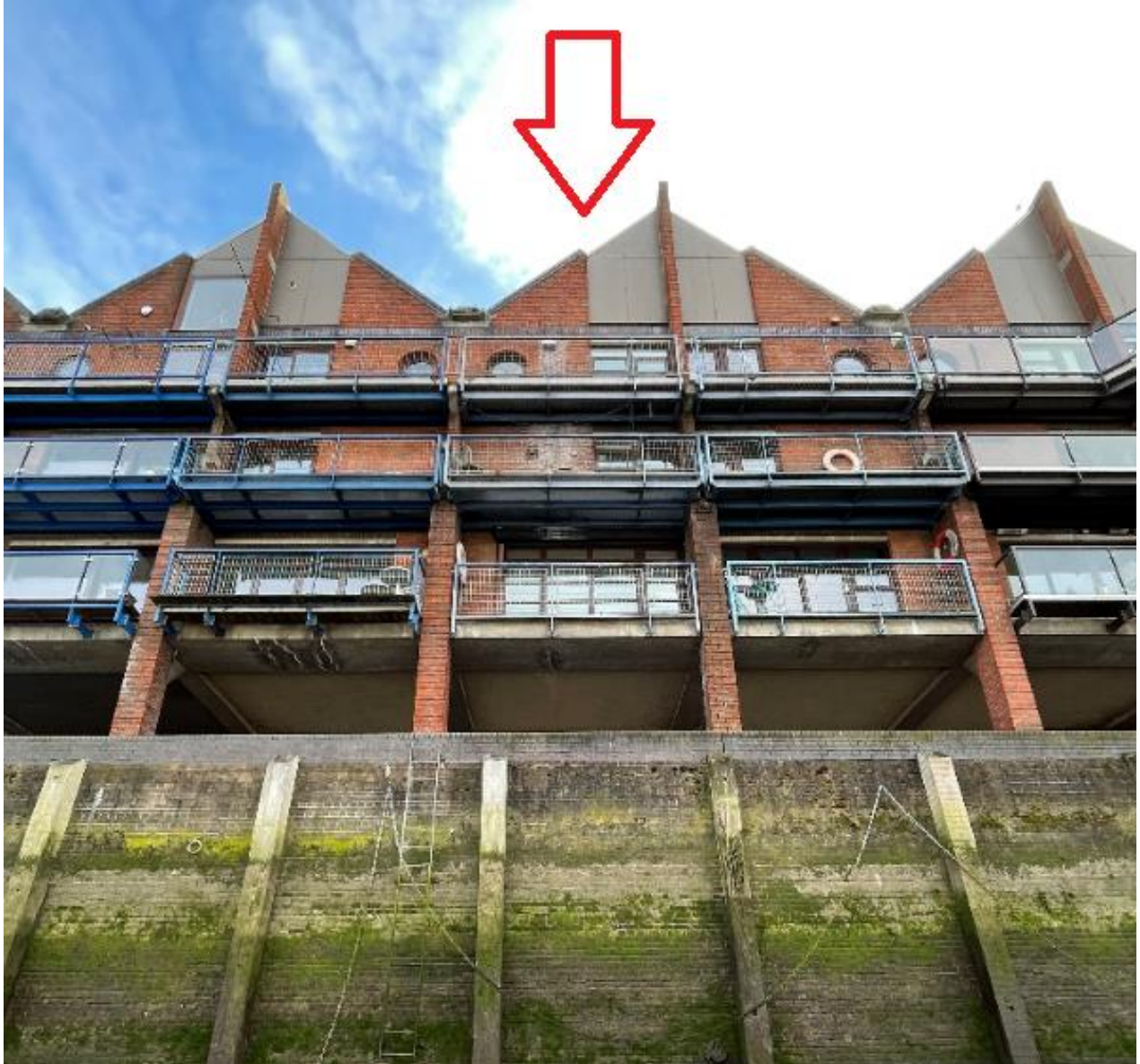
9 Kings Stairs Close (arrowed in red) – North Elevation
