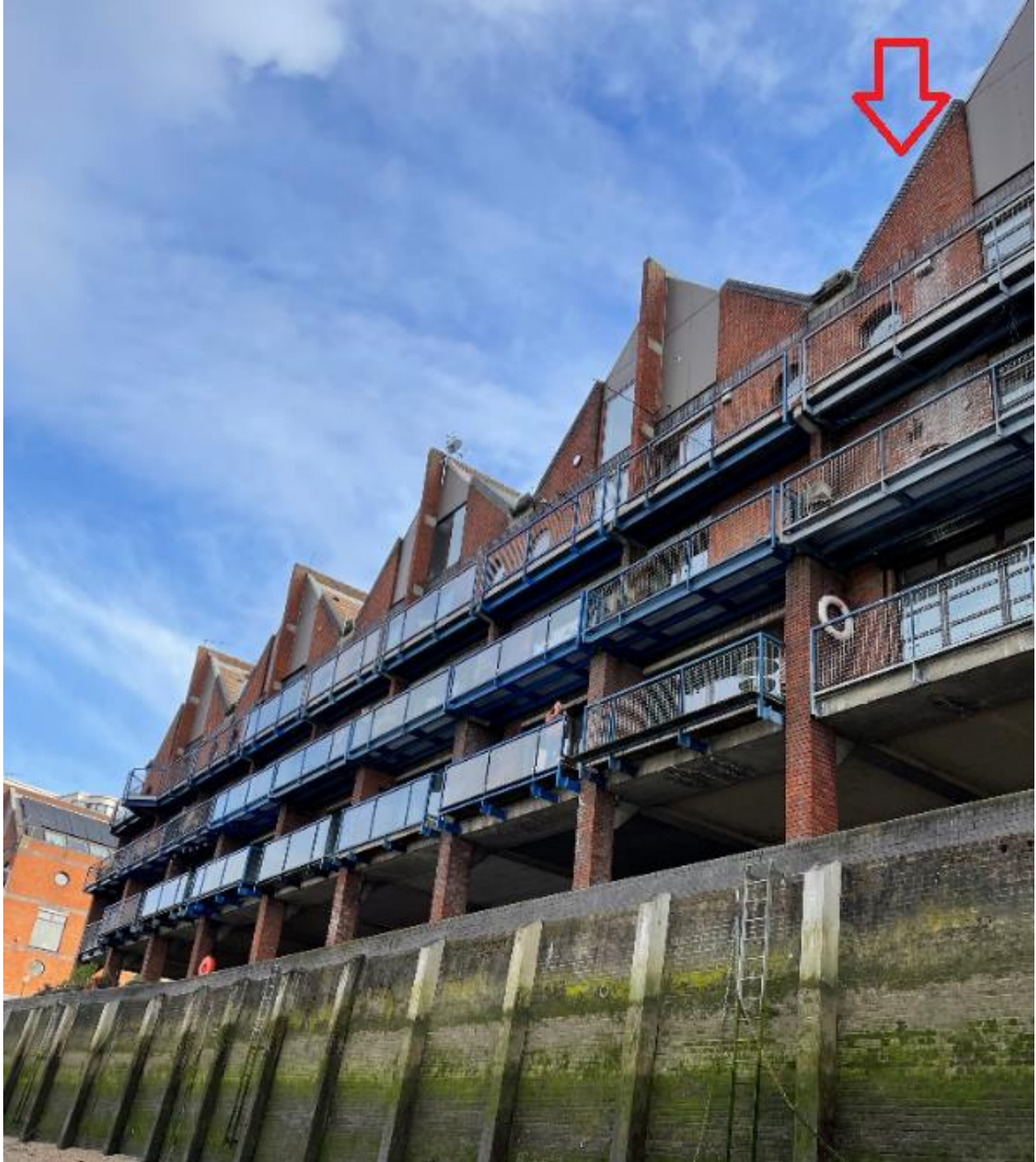
9 Kings Stairs Close (arrowed in red) – North Elevation
