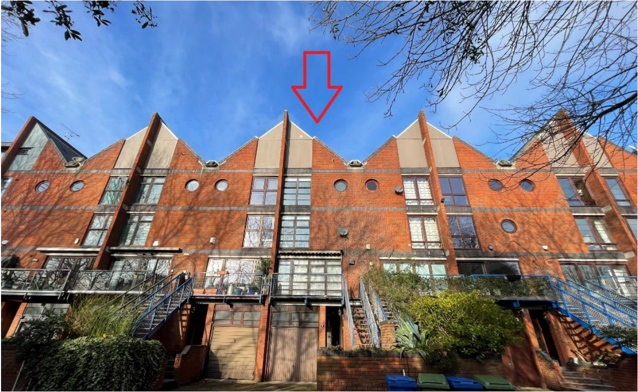
9 Kings Stairs Close (arrowed in red) – South Elevation
