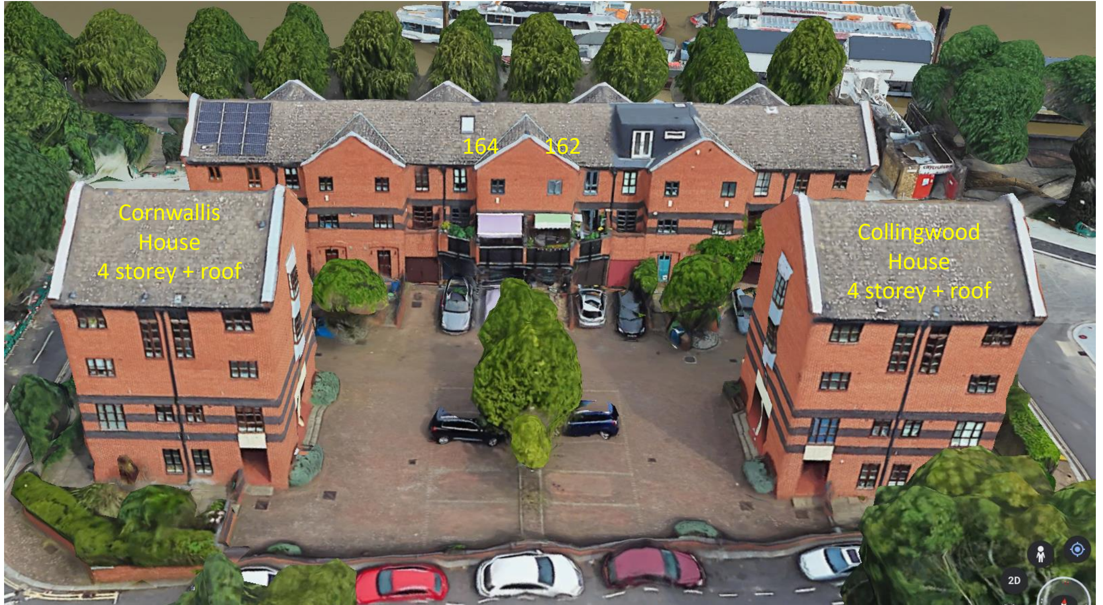
REAR VIEW OF 162 AND 164 BERMONDSEY WALL EAST
