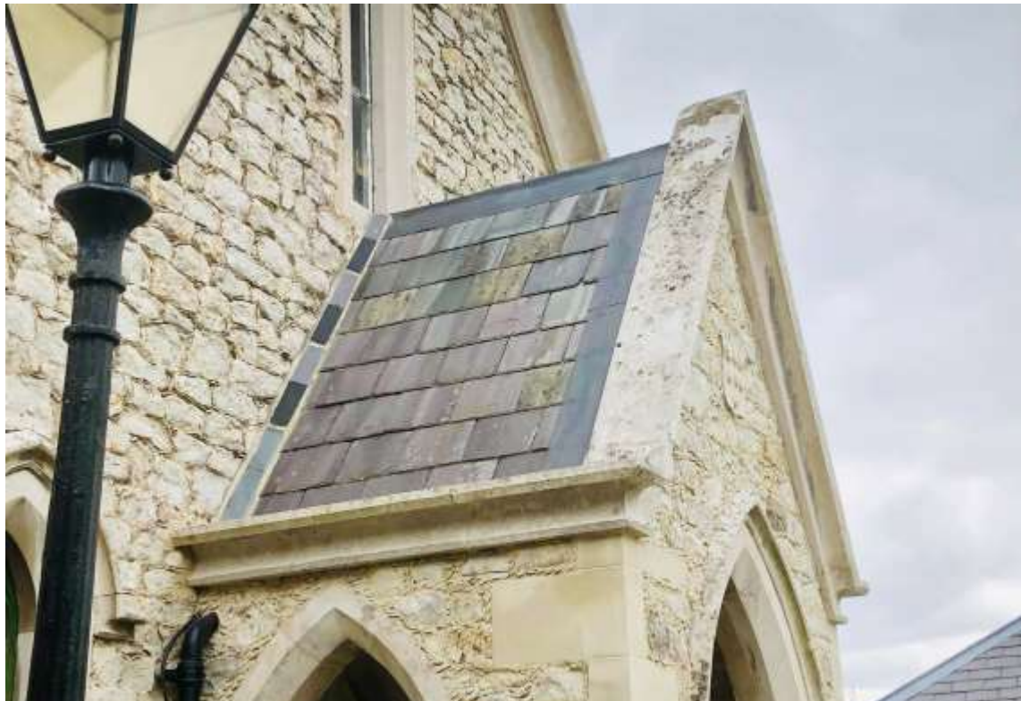
Fig 3: The Grade II listed building dates from the mid-19 th Century and uses galleted roughly coursed rubble with stone quoins, a gable end central attic and porch with two low pitched hipped side wings topped in slate.
