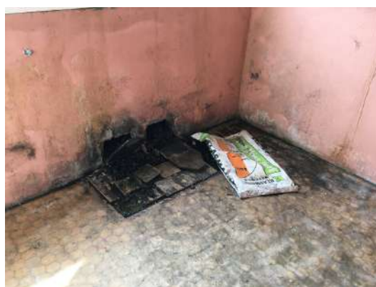
Photograph 4. Access to coal bunker in outbuilding.
