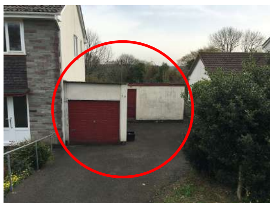
Photograph 1. North elevation. (survey area outlined in red)
