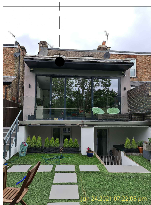
Rear of No.286 Ballards Ln
