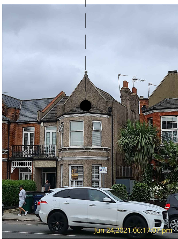
Front of No.286 Ballards Ln
