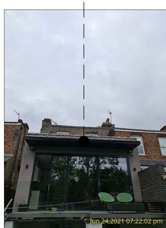
Rear of No.286 Ballards Ln
