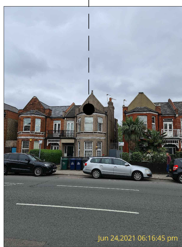
Front of No.286 Ballards Ln
