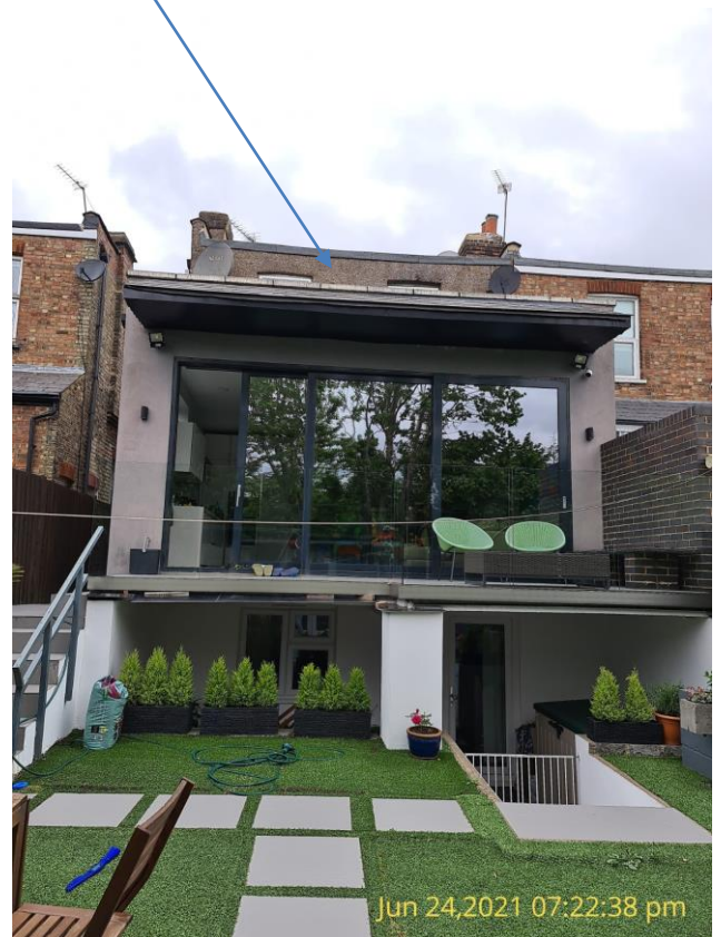
Application Site – Rear View
