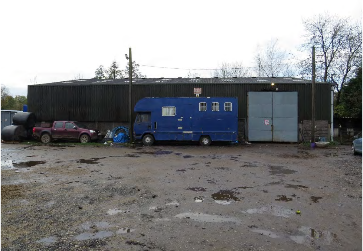
1 – Building 1 is a large steel agricultural building.
