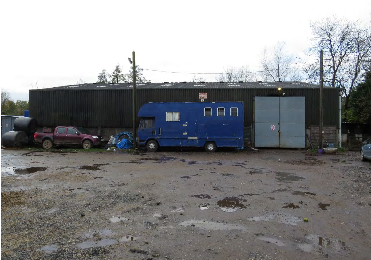
3.1a – The east side of building 1 viewed from the south.
