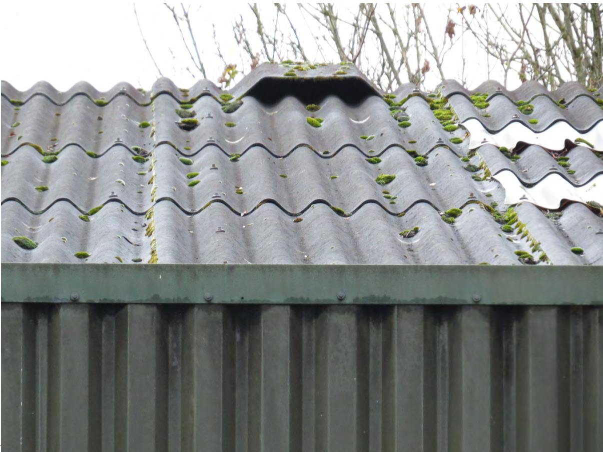
2 – The walls and roof are corrugated steel and corrugated asbestos cement.
