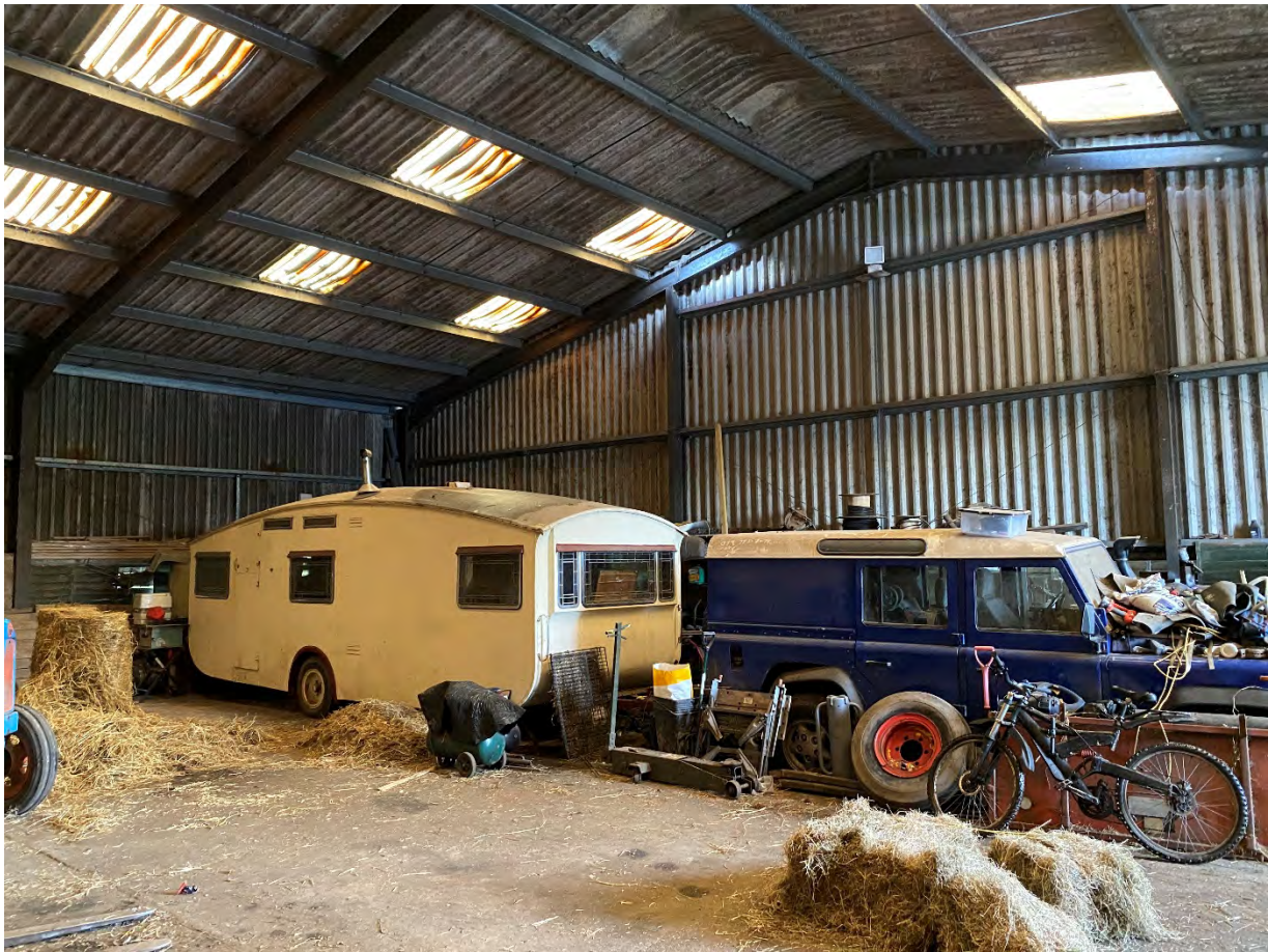
3.2a – The inside of the barn.
