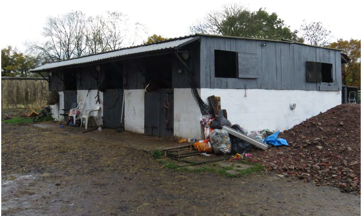
5 – All stable blocks have a similar construction.
