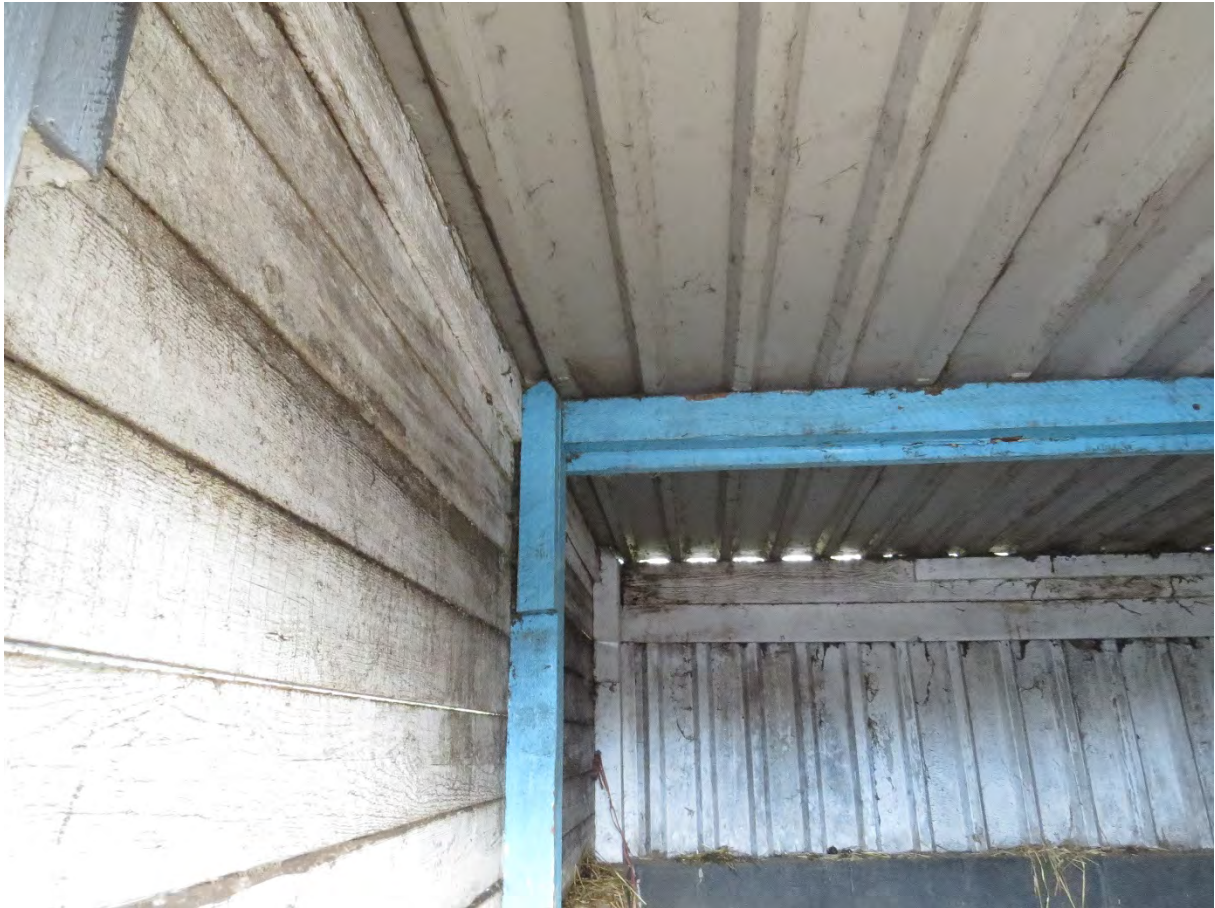
7 – Roofs have a simple timber structure with sheet metal coverings.
