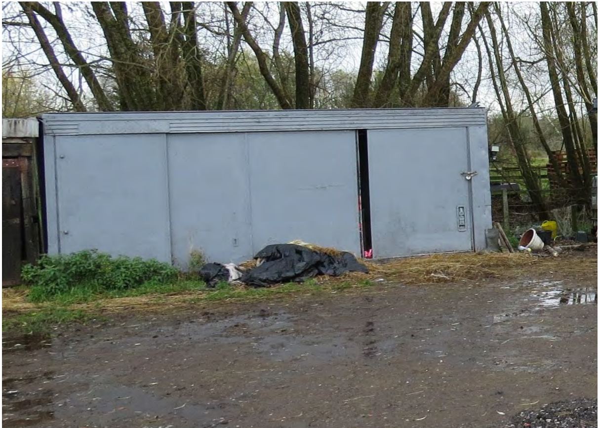
8 – Building 8 is a steel storage container with no suitable features.
