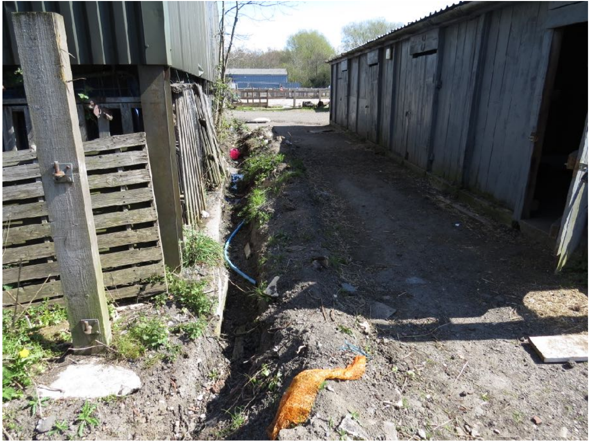
9 – The ditch takes drainage and runoff from the site.
