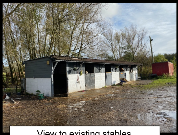
View to existing stables
