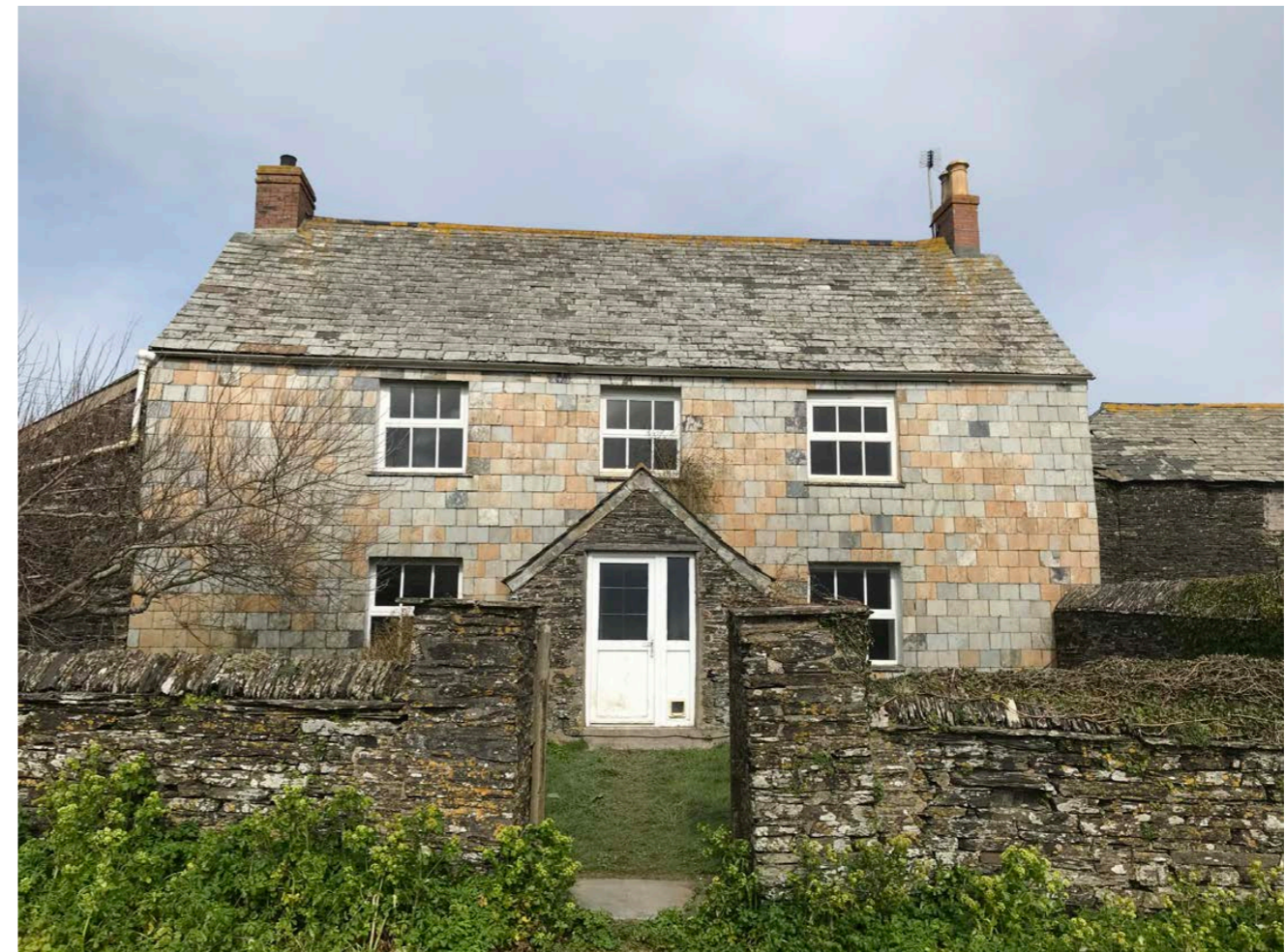
South Elevation of Porthmissen Farmhouse
