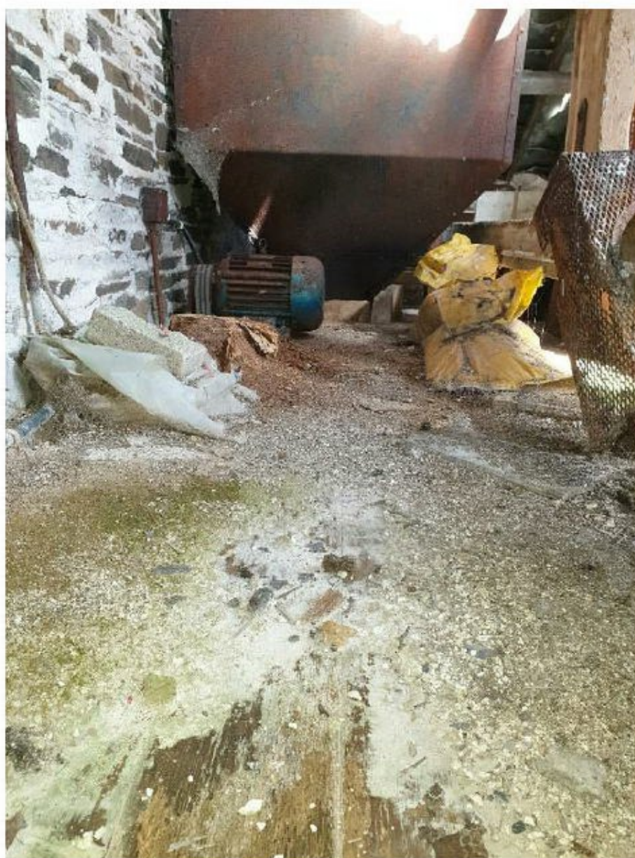
Figure 13: Mezzanine floor at western end of single-storey section of Barn 1 (viewed towards the north)
