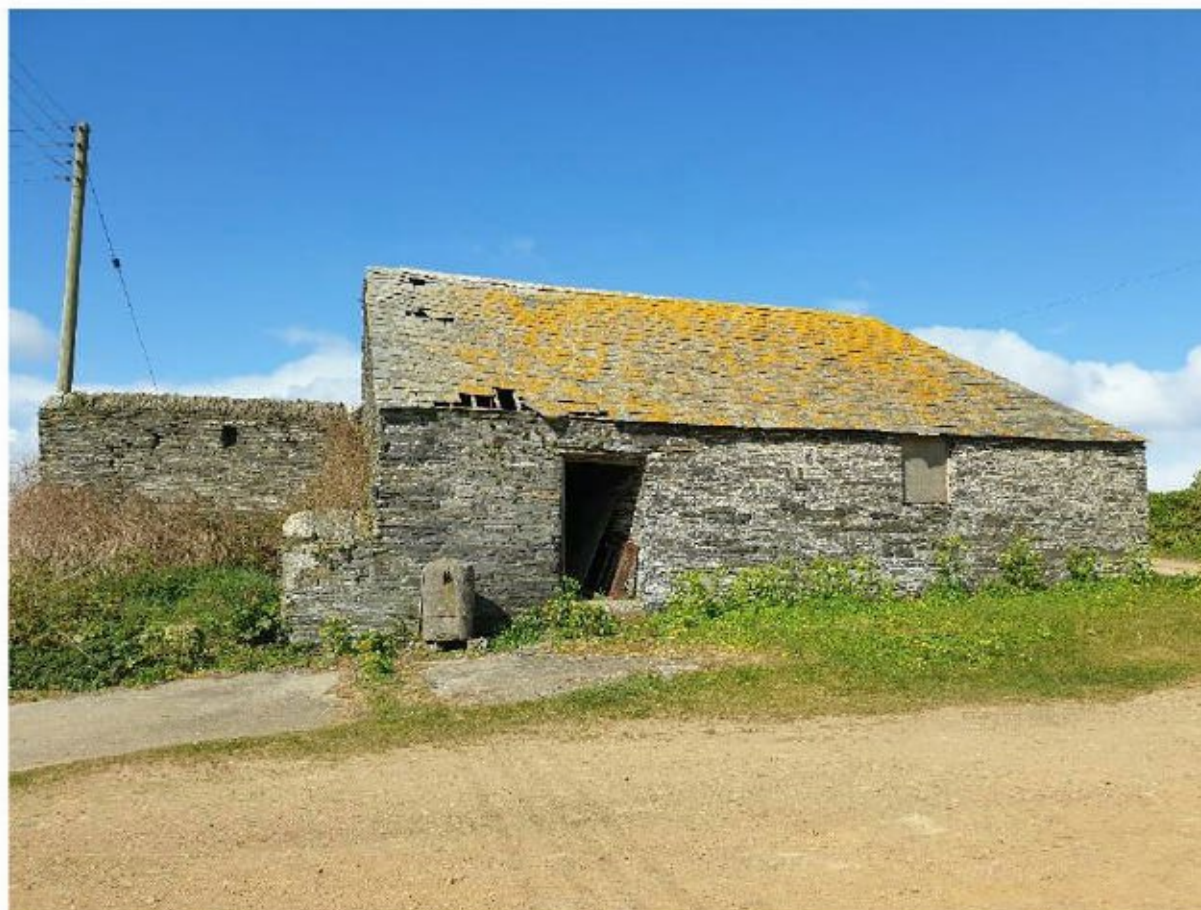
Figure 21: Eastern elevation of Barn 3 at Porthmissen Farm
