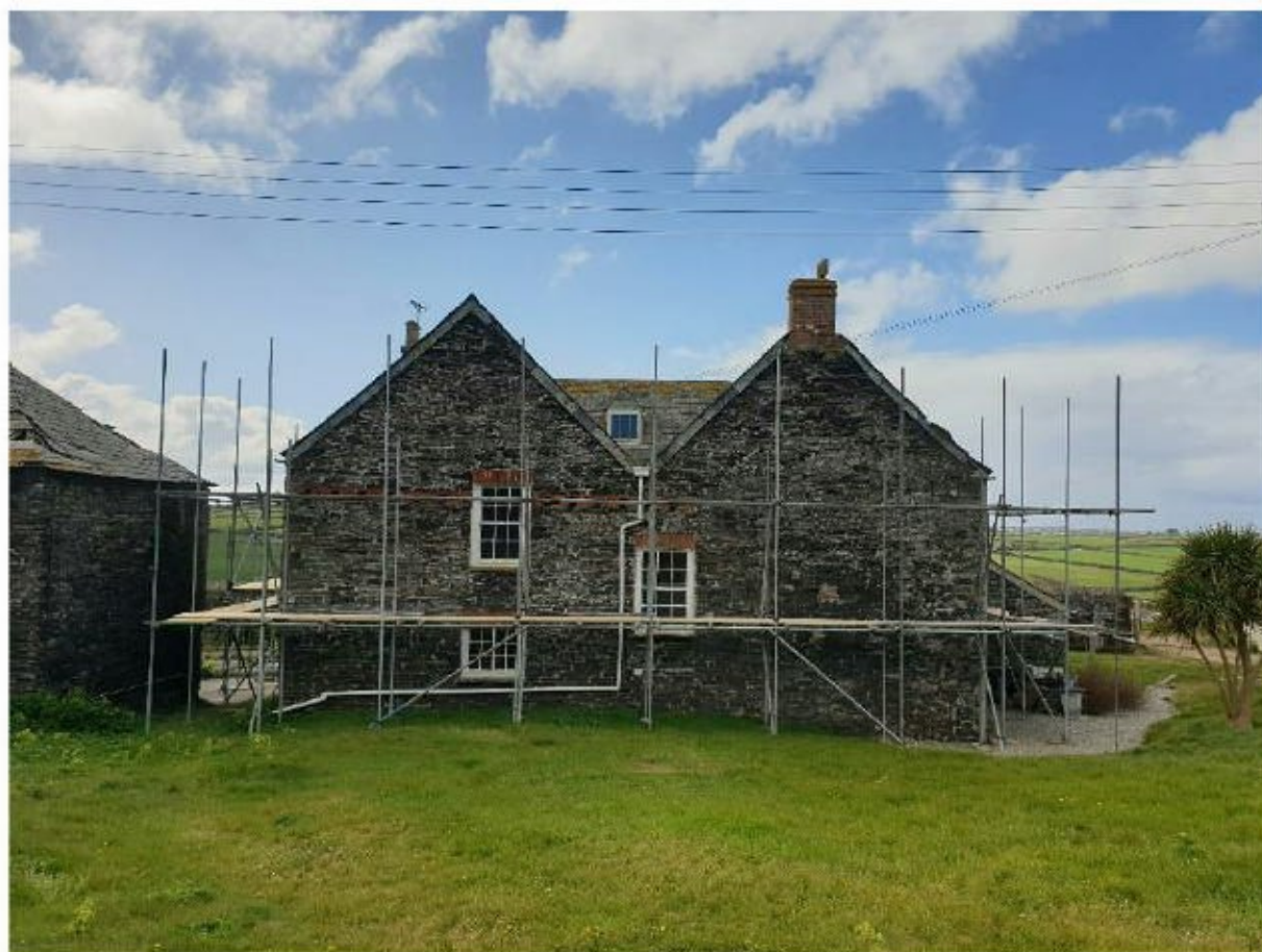
Figure 3: Northern elevation of farmhouse at Porthmissen Farm
