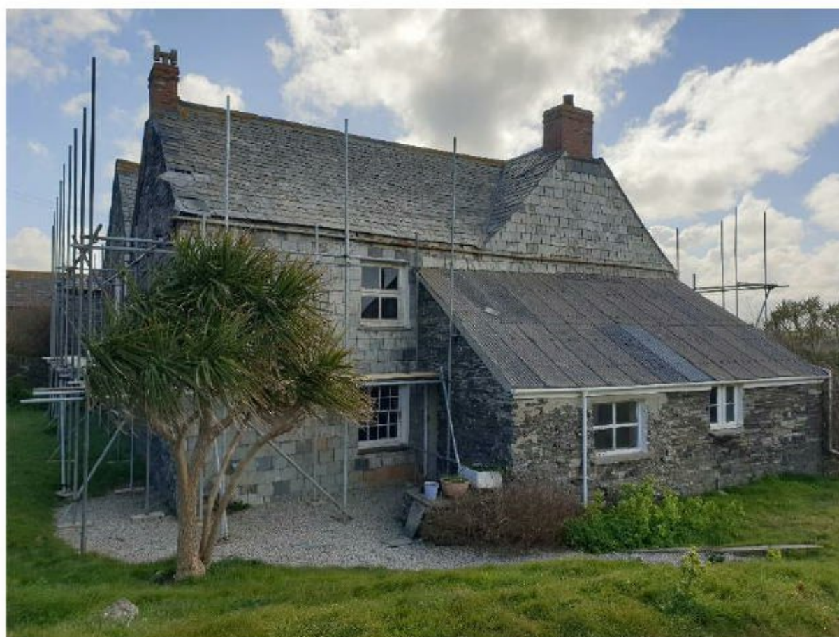
Figure 4: Western elevation of farmhouse at Porthmissen Farm
