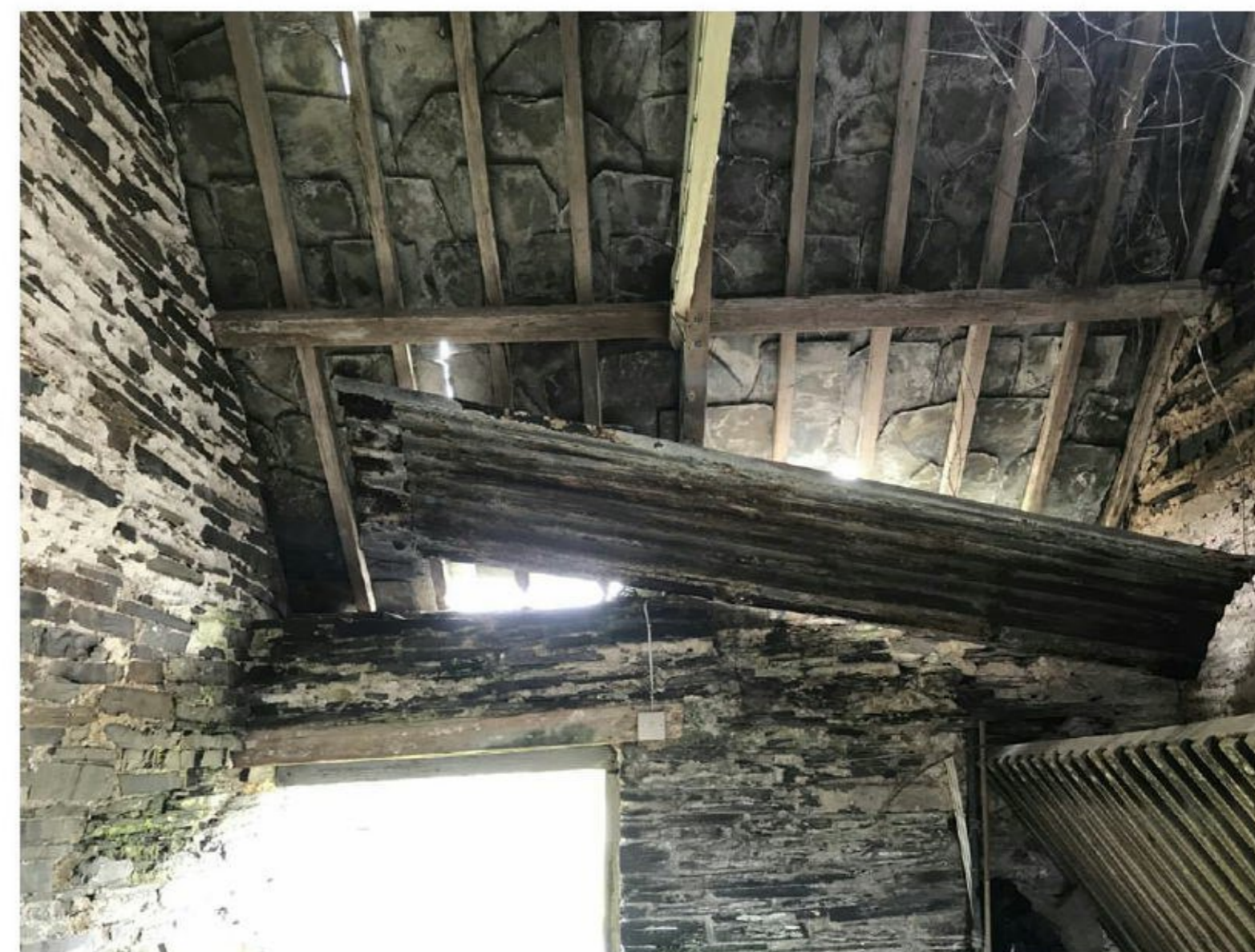
Left - View of underside of rag slate roof showing structure
