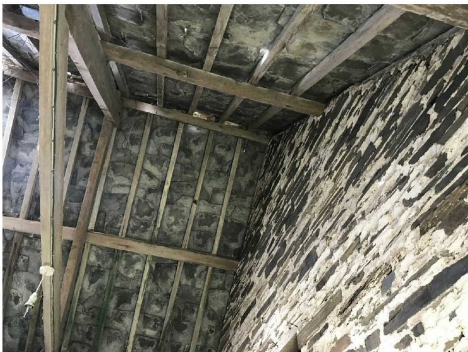
Left - View of underside of rag slate roof showing structure
