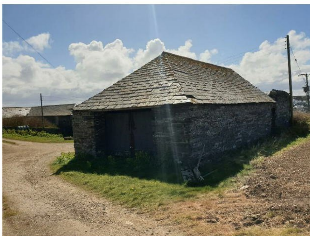
Figure 22: Northern and western elevations of Barn 3 at Porthmissen Farm
