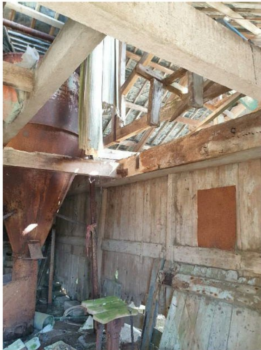
Figure 12: Interior of single-storey section of Barn 1 (viewed towards the north)
