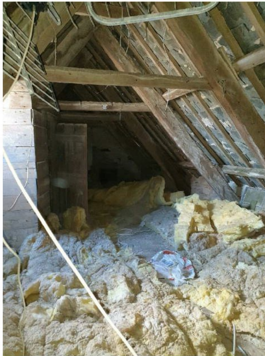
Figure 7: Interior of southern roof void (viewed towards the east)
